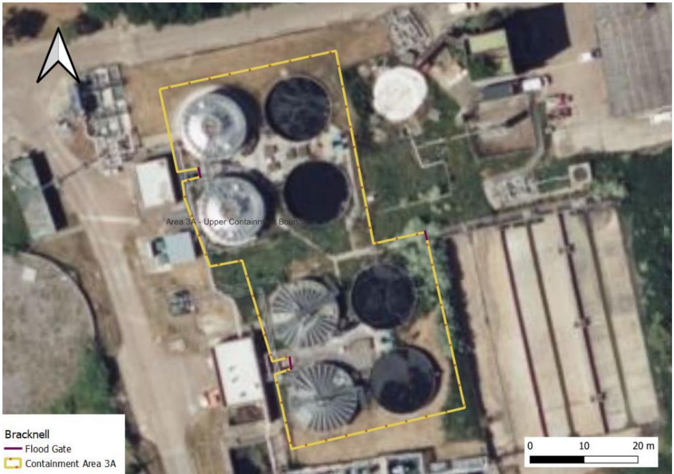
Figure 15 - Containment Area 3A – Close Containment Area
