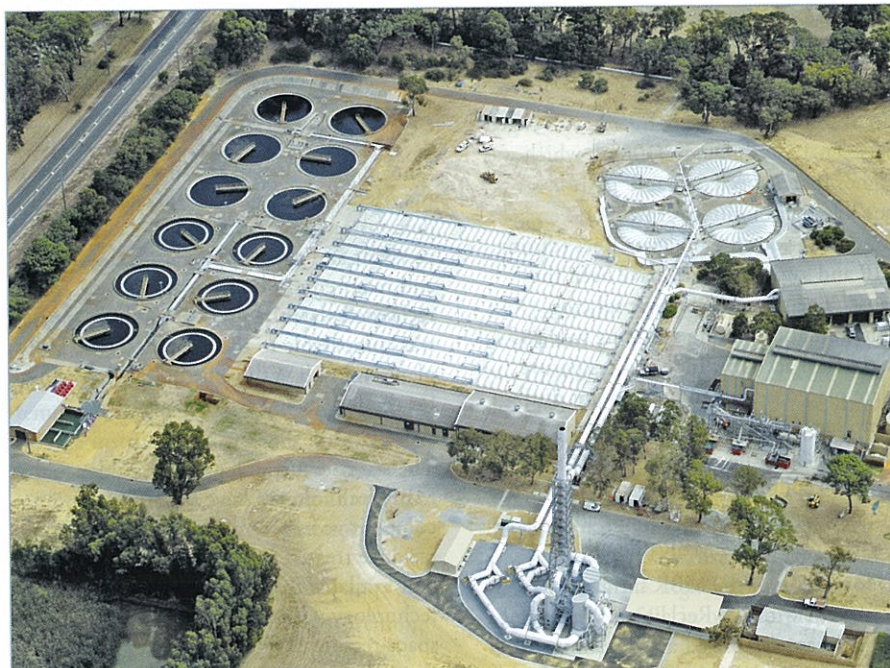
Figure 1. Subiaco Wastewater Treatment Plant.
