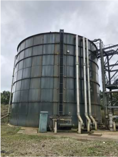
Photo 4 – Unthickened sludge storage tank
