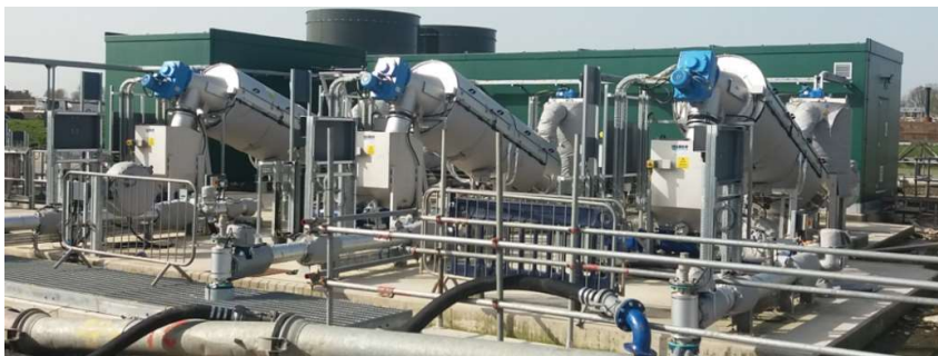
Photo 1 – Drum thickeners (x3)
