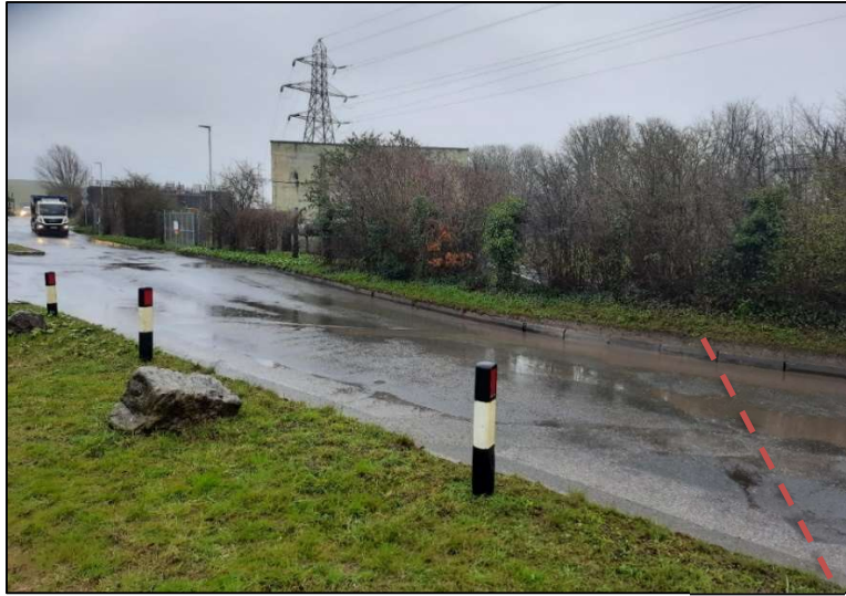
Plate 3.7.3: The Ride showing the approximate location of the below ground route of the discharge channel (dashed red line)
