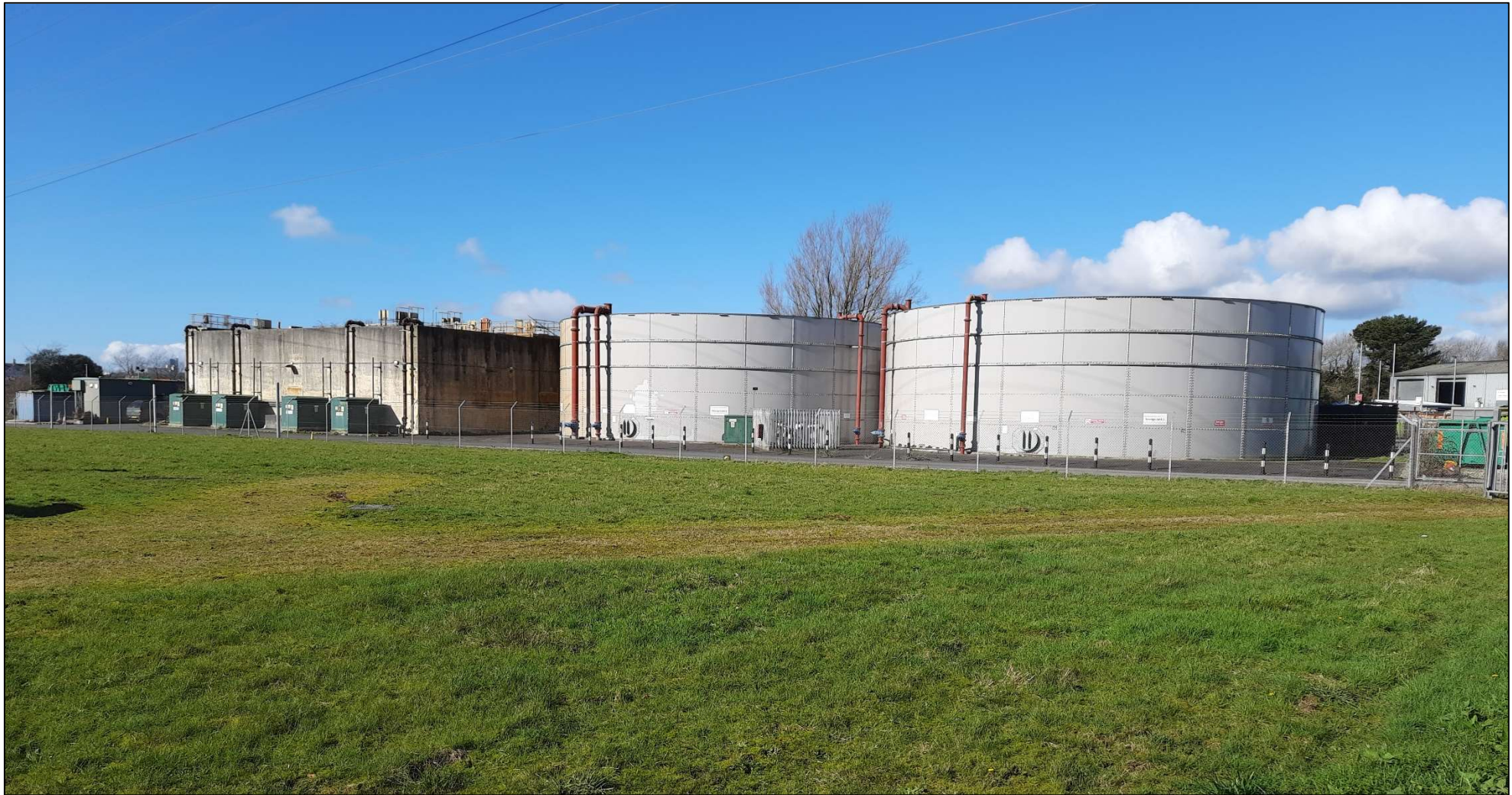
Plate 1.6: Leachate Treatment Plant, looking south west from the lagoon pumping station, Chelson Meadow, Plymouth 2021. Infrastructure components from left to right are: Sequential Batch Reactors (SBRs), STOR 2 & STOR 1
