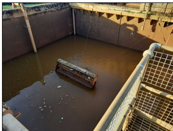
Plate 5.6: Source SBR3 in the post-decant period, before blowers are activated and available as a source of liquor
