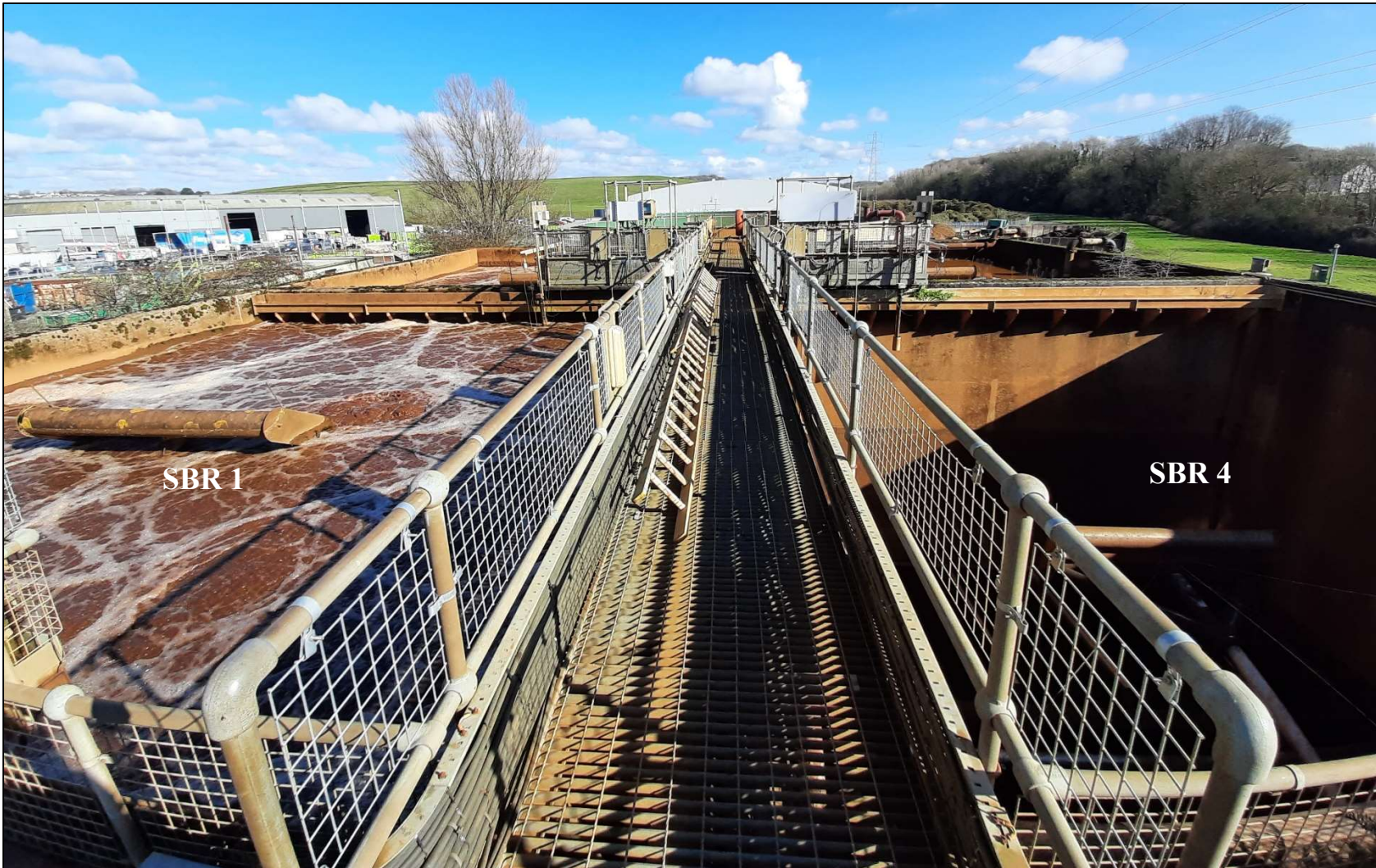
Plate 3.4.4: Looking east across the top of the walkway serving the SBRs, 2021
