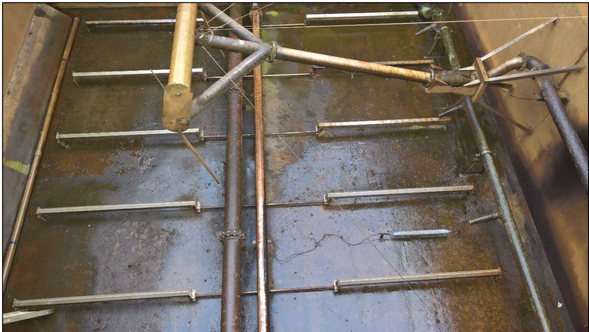
Plate 5.21: Cleaned SBR ready for any required servicing or repairs
