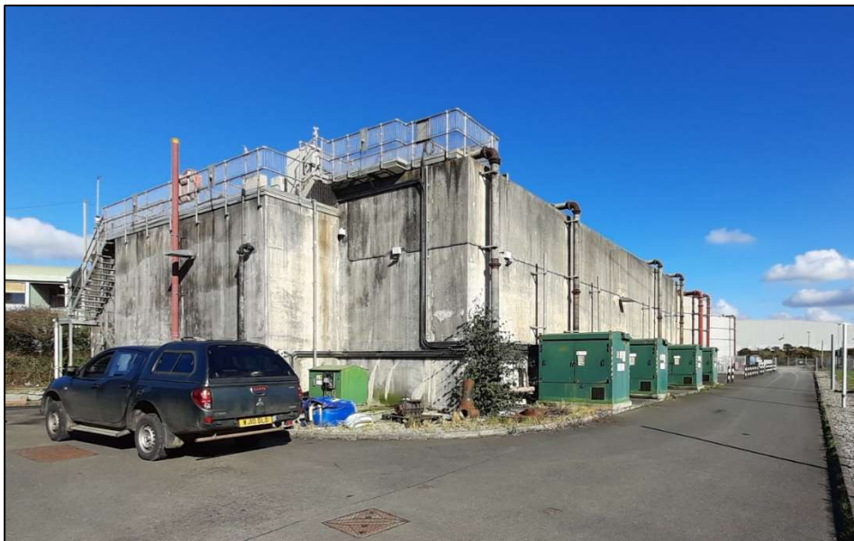
Plate 3.4.1: External view of SBR plant, 2021
