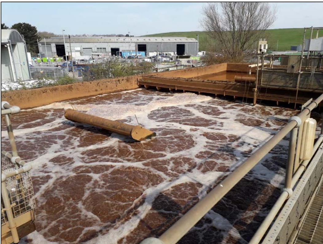
Plate 1: SBR 1 in the react phase and suitable for the collection of a Mixing/Aerating sample
