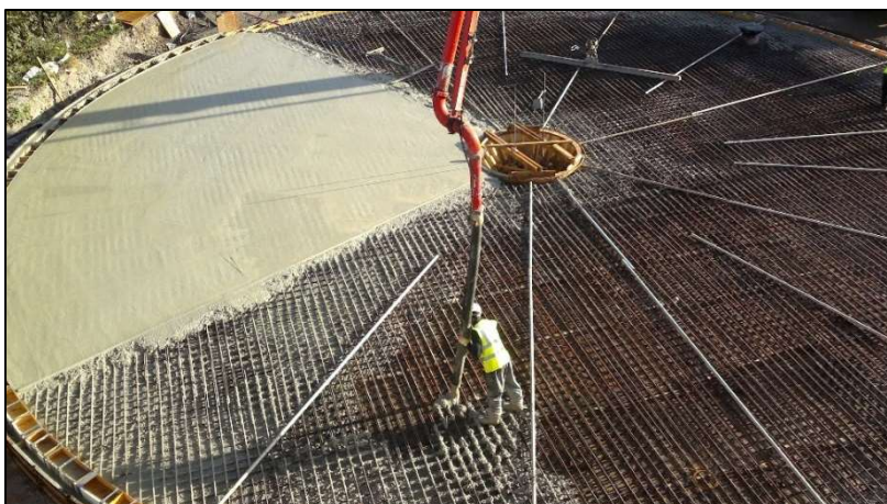
Plate 3.1.2: Laying concrete for the base to STOR2
