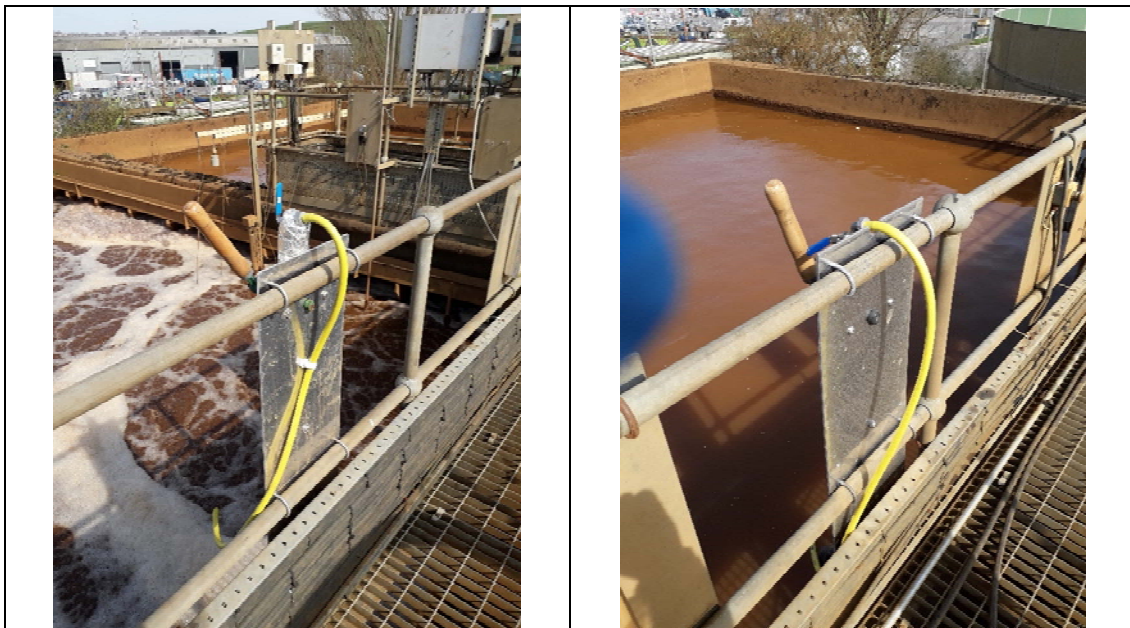
Plate 3: Manual sampling pump in SBR
