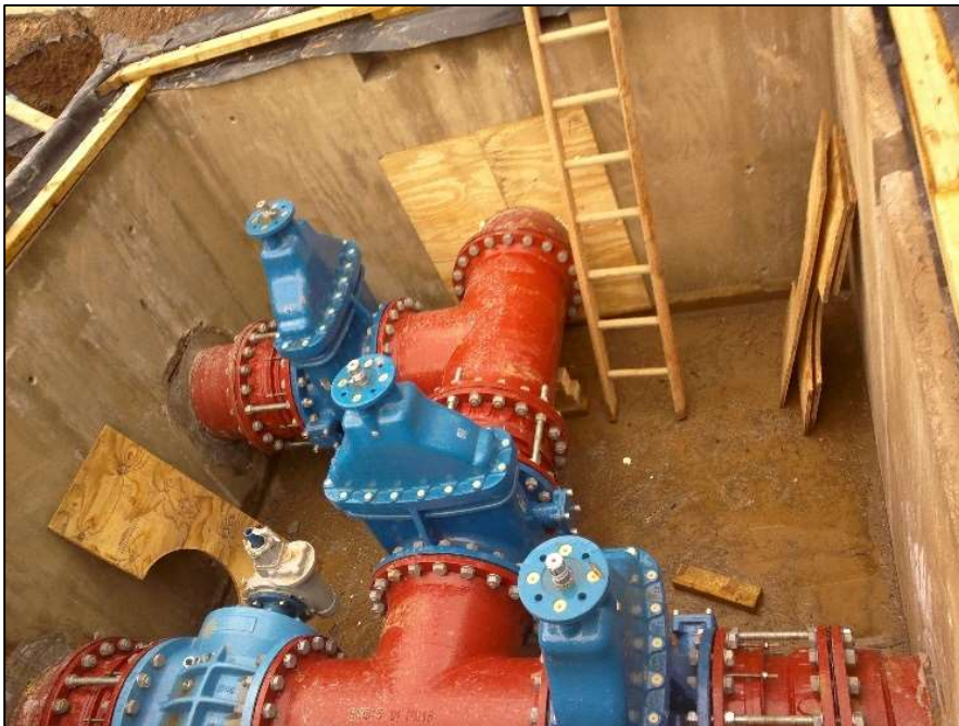
Plate 3.2.2: Installation of valves to STORs 1 & 2
