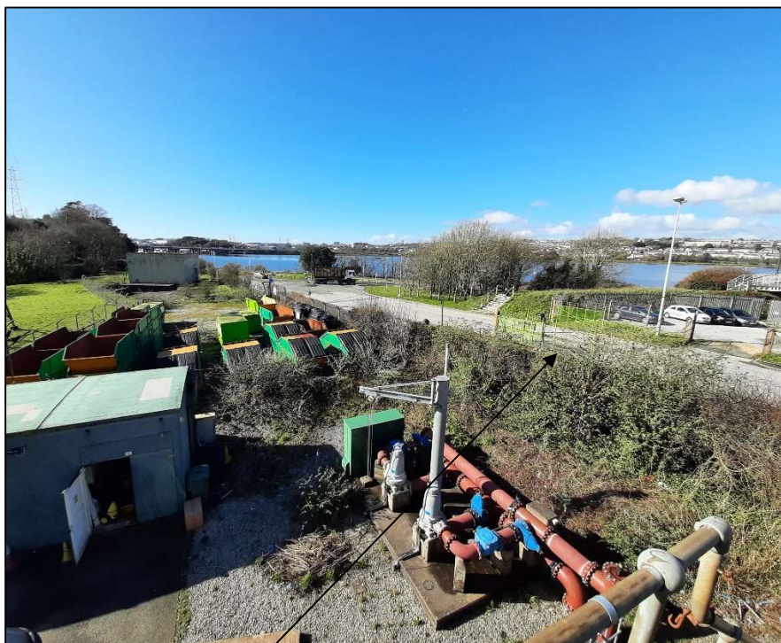
Plate 1.11: Section of security fence surrounding the LTP (obscured by vegetation), looking west from the top of the SBR 2021
