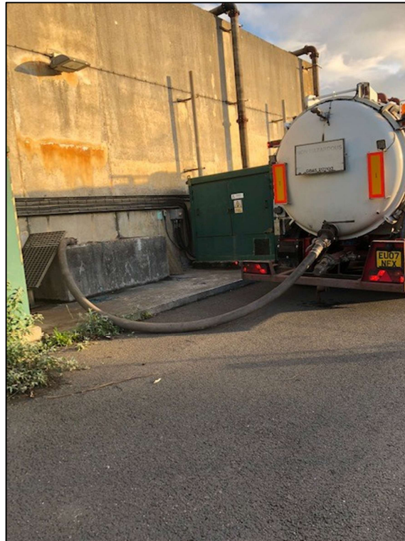
Plate 5.20: Tanker emptying the outlet sump during cleaning of the SBR
