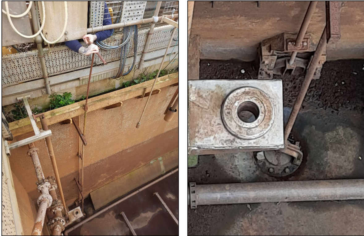
Plate 5.17: Outlet point being opened (left) and left open (right) throughout cleaning of SBR
