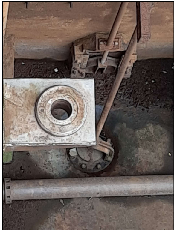
Plate 5.11: Manual closure of outlet point from SBR
