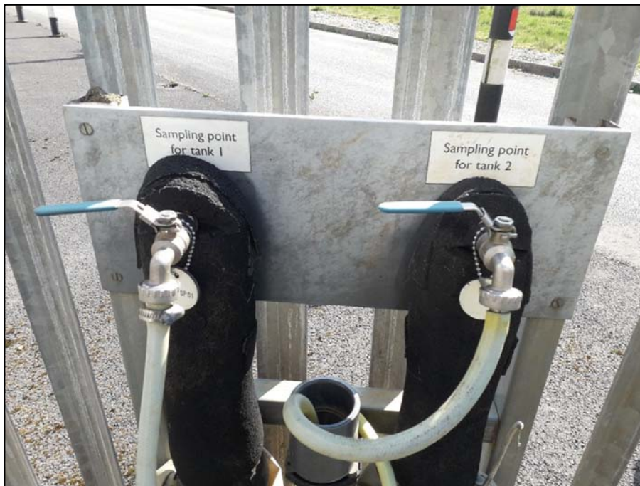
Plate 13: Sampling points for STOR1 and STOR2 inside the actuated valve cage
