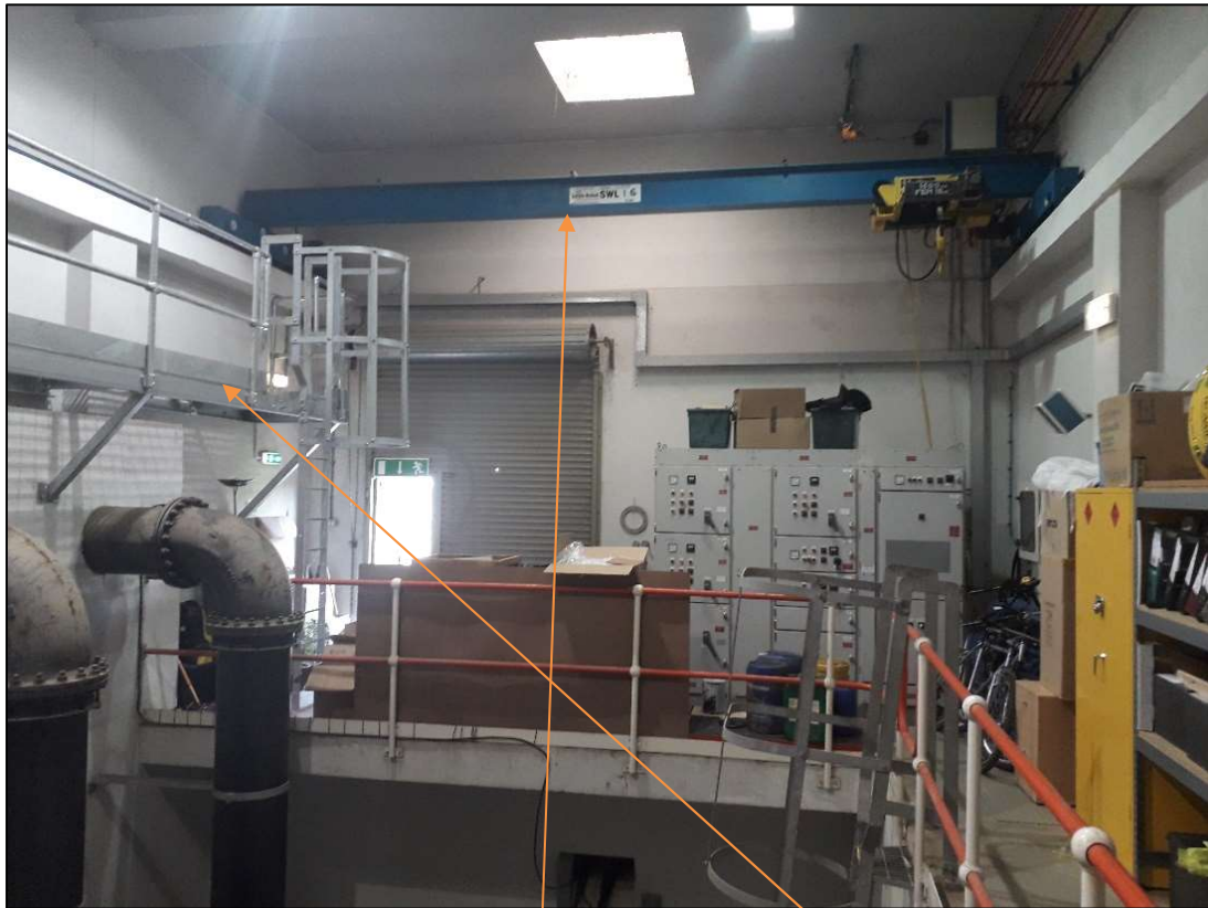
Plate 3.3.5: Overhead crane and gantry for crane inspection
