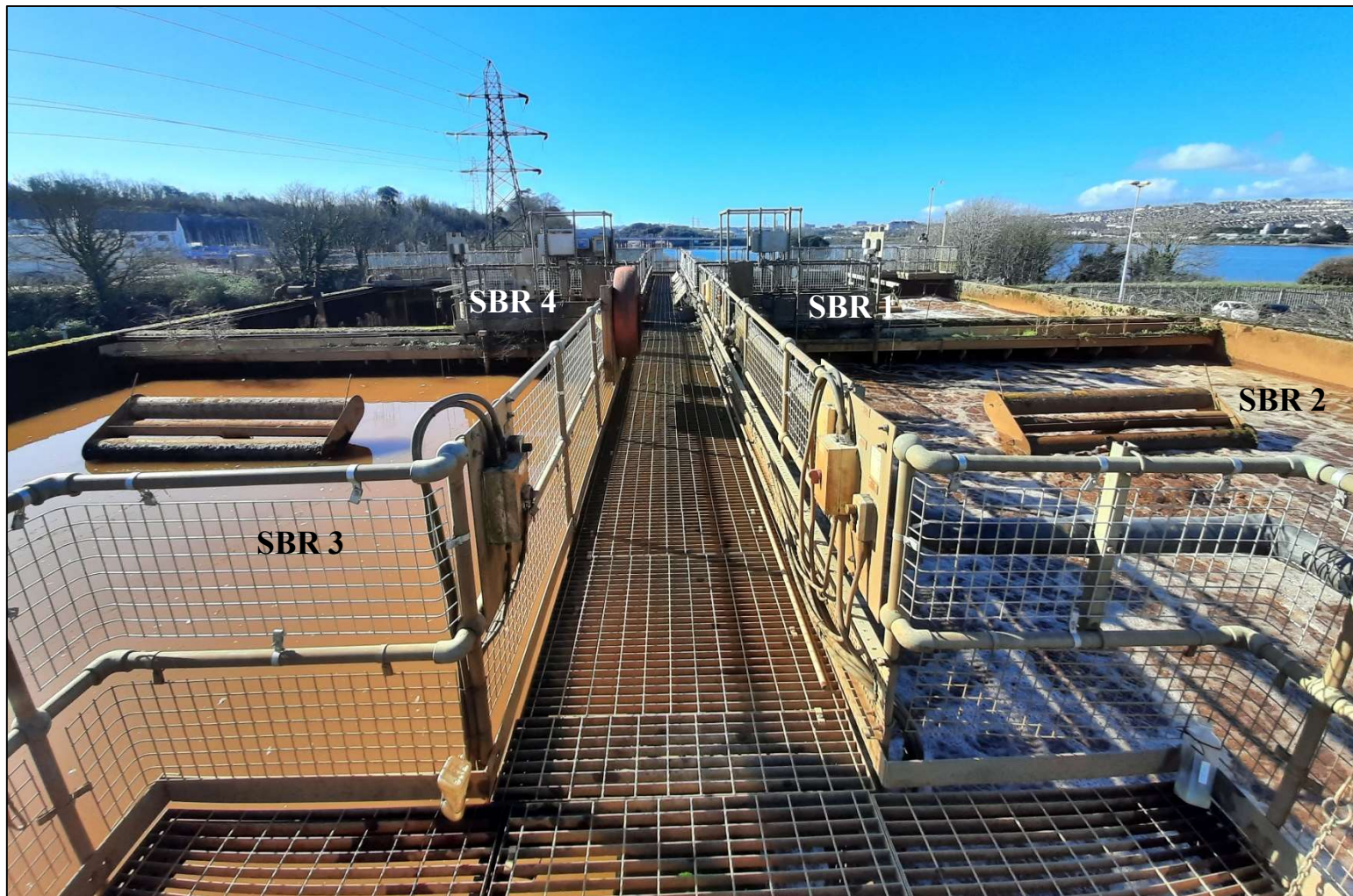
Plate 3.4.3: Looking west across the top of the walkway serving the SBRs, 2021
