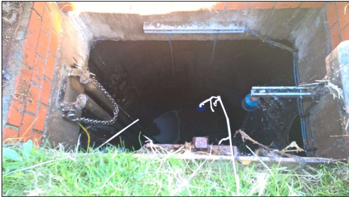
Plate 2.19: Looking into the Lagoon leachate well, showing the pump and associated infrastructure, August 2018
