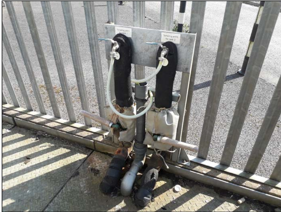
Plate 12: Sampling points for STOR1 and STOR2 inside the actuated valve cage
