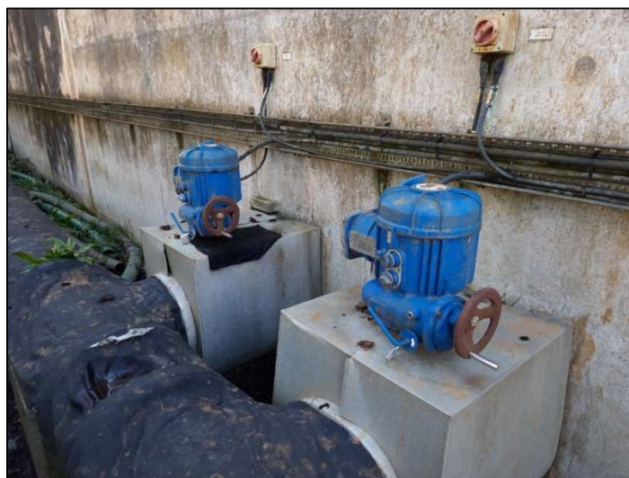
Plate 3.4.6: Two inlet valves, one serving SBR1 and one serving SBR4
