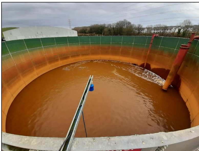
Plate 5.3: STOR1 containing raw leachate derived from throughout the landfill, 2021
