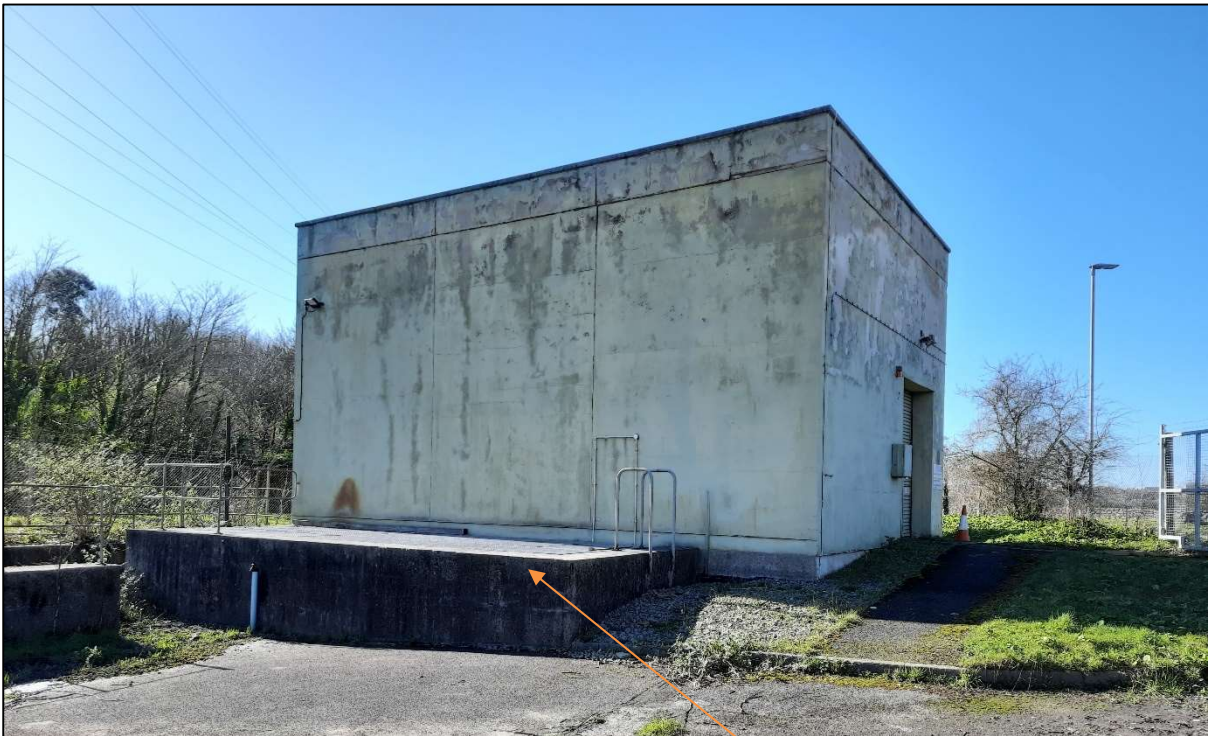
Plate 3.3.1: Pump lifting station & wet well, 2021
