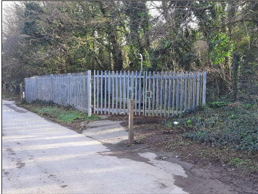
Plate 1.12: The Ride pumping station, viewed from the Ride, 2021
