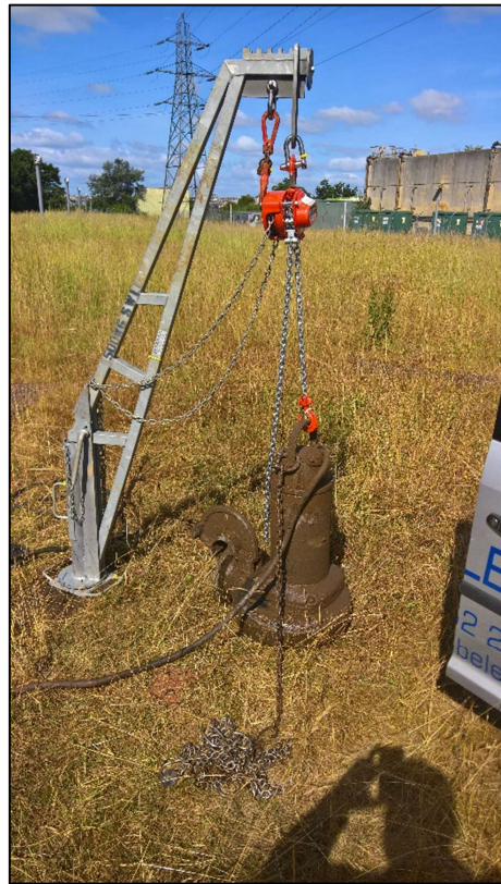
Plate 4.1.6: Removal of Lagoon Pumping Station leachate well manhole cover, and raising of pump therein
