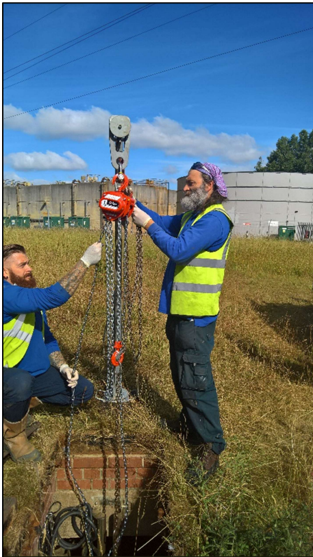
Plate 4.1.6: Removal of Lagoon Pumping Station leachate well manhole cover, and raising of pump therein
