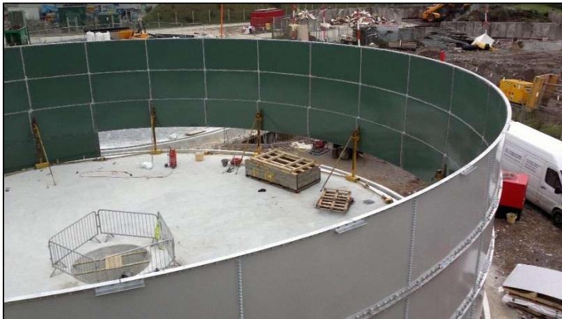
Plate 3.1.4: Construction of glass-coated steel tank sides to STOR2
