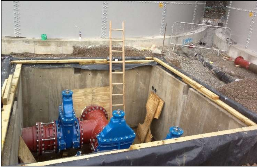
Plate 3.2.1: Installation of valves to STORs 1 & 2
