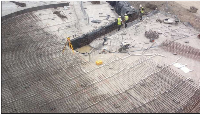
Plate 3.1.1: Preparation of the reinforced concrete slab for the new STOR2
