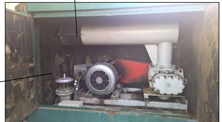
Figure 3.4.7: Illustrated cross-sectional plan of SBR external infrastructure (blowers)
