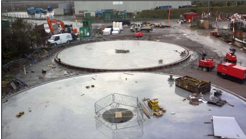
Plate 3.1.3: Completed concrete base to STOR1 and STOR2
