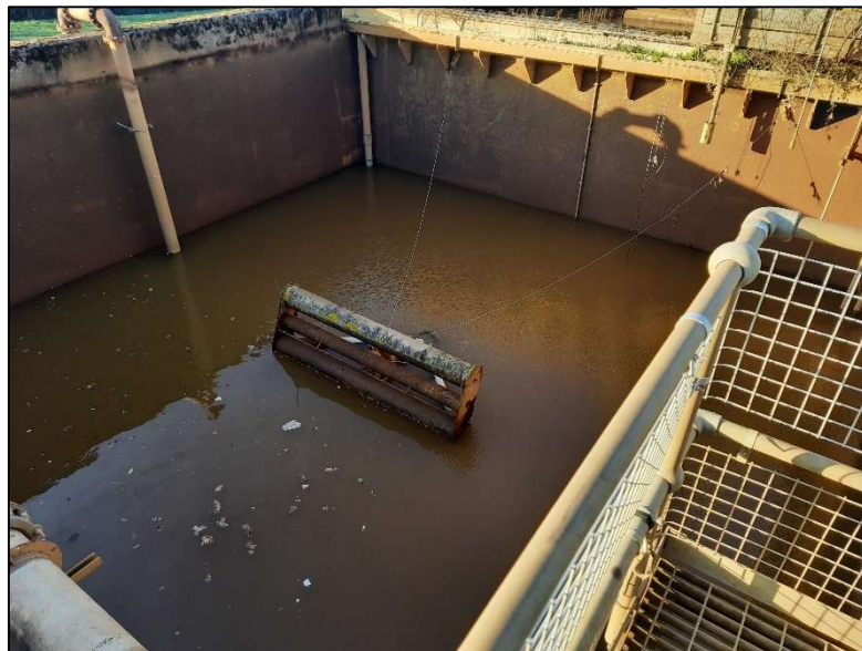
Plate 5.4 Leachate-receptive SBR containing treated leachate and bacterial biomass (mixed liquor), 2021
