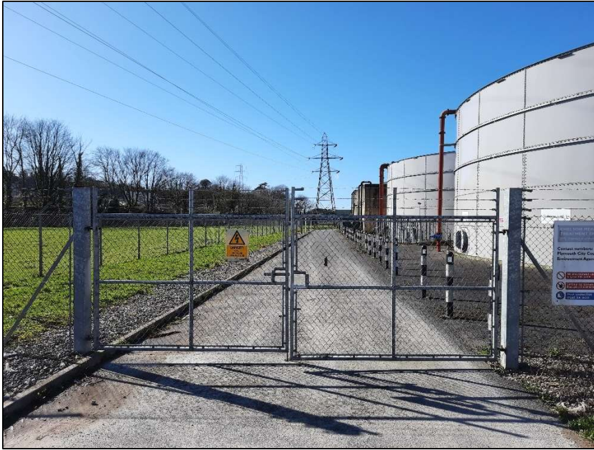
Plate 1.8: Security gate to the LTP, looking west from the site entrance 2021
