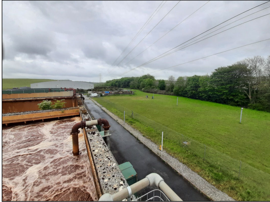
Plate 1.3: Southeast boundary to the permit area, looking southeast across the old lagoon towards the new residential development, viewed from the top of the SBR, 2021
