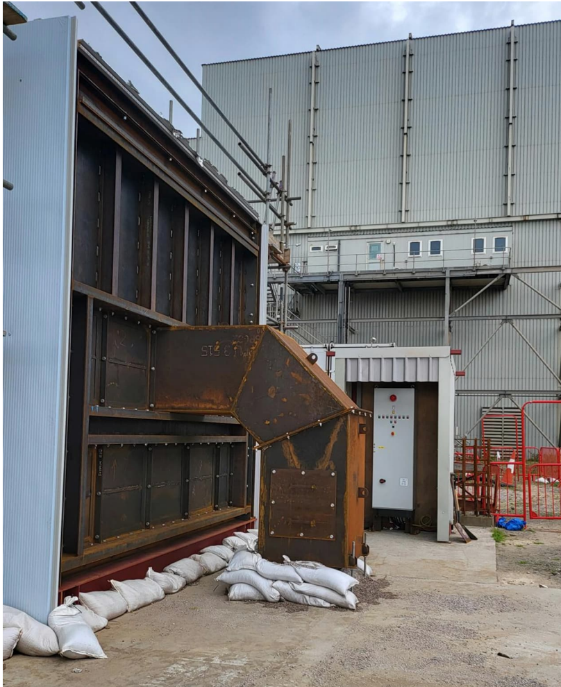
Figure 5-14 - Acoustic Enclosure with Material Discharge Chute
