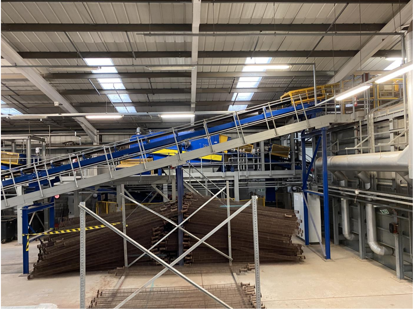
Photograph 13: Conveyors inside processing building. Hard standing in good condition.
