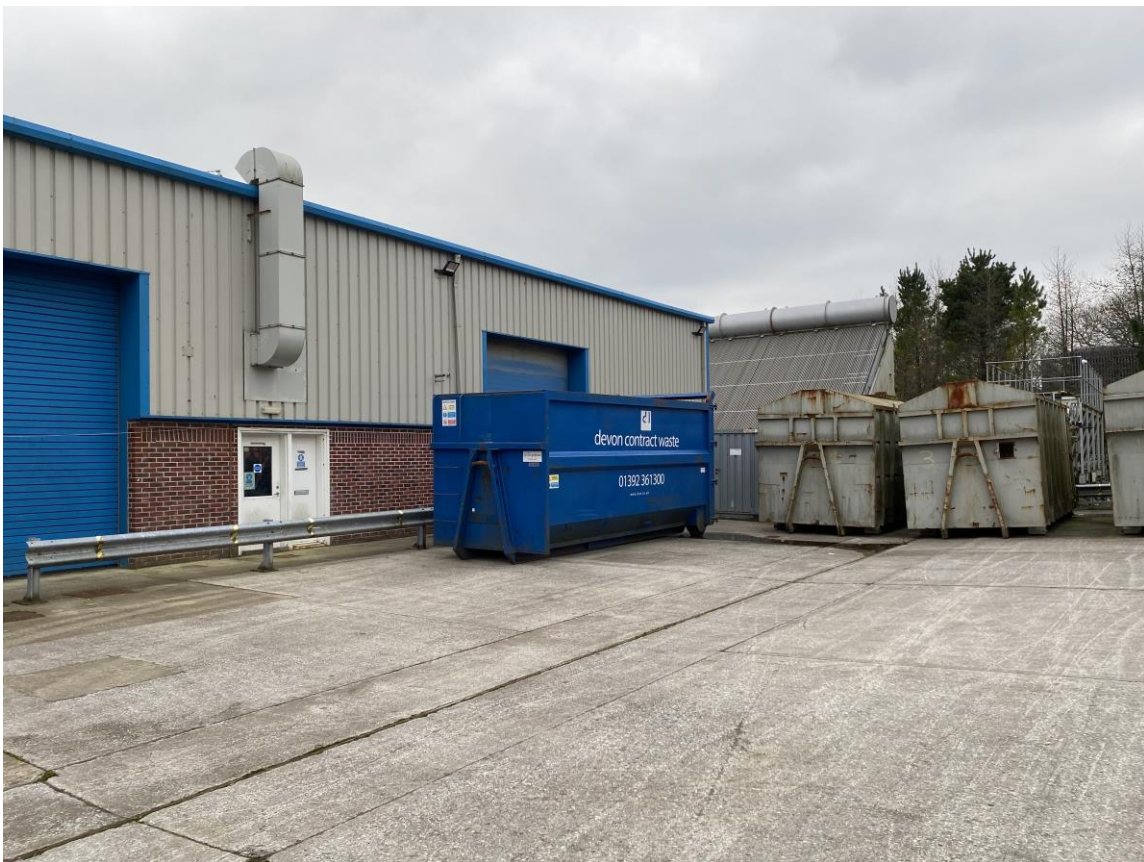
Photograph 8: View of northwest corner of the site from the main yard.
