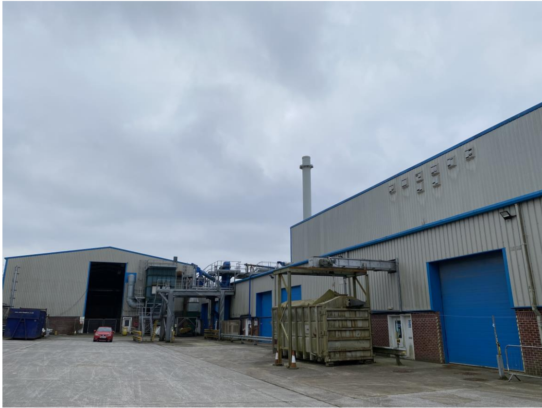
Photograph 9: View of facility looking south from the main yard. Reception hall is to the left of the image and stack visible in background.
