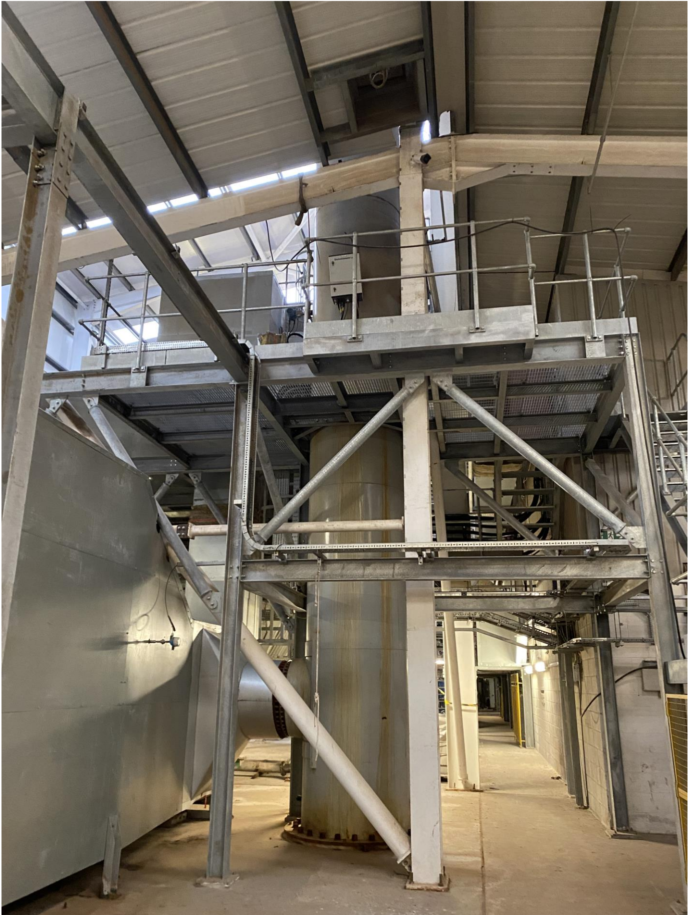
Photograph 14: View of stack from inside the building.
