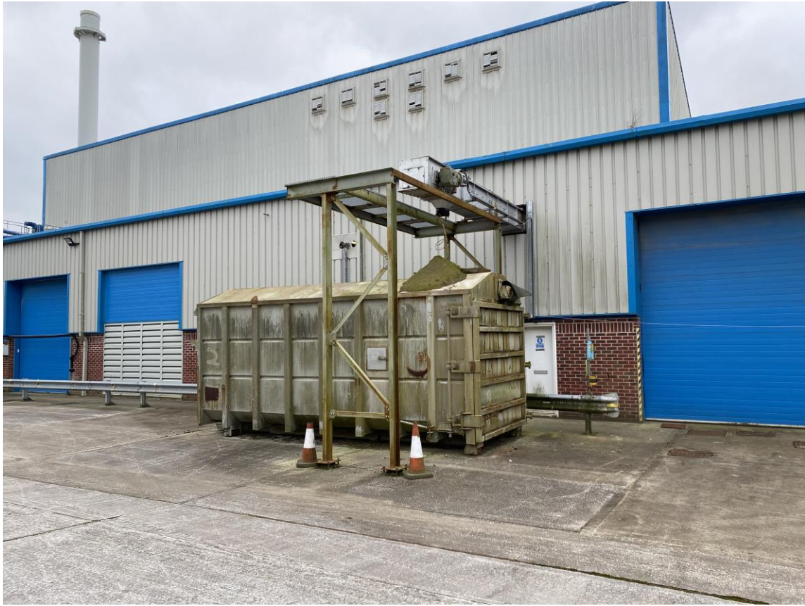
Photograph 7: View of northeast side of the building from main yard.
