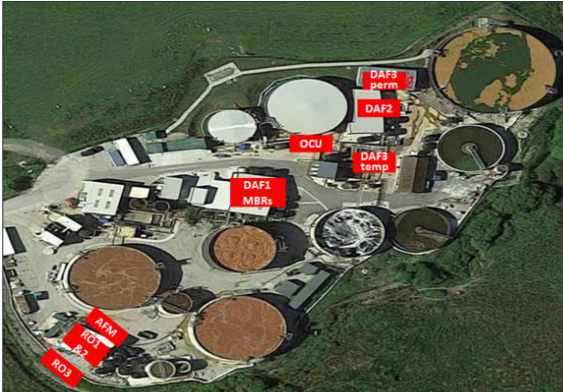
Figure 4-23 – Location of DAF1 / DAF2 / DAF3 at the WPF (and other plant & equipment)
