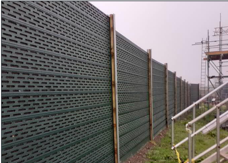
Figure 5-5 – Photo of Acoustic Fencing Installed
