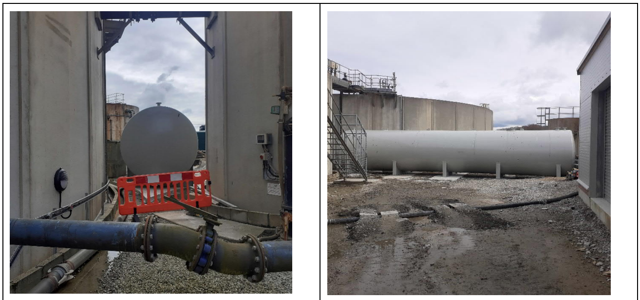
Figure 4-27 – Photos During Installation of UF / RO Flow Attenuation Tank
