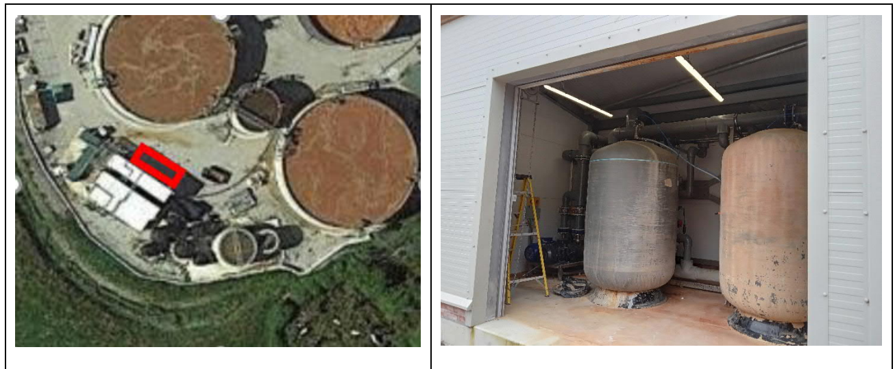
Figure 4-25 – New AFM Tanks Location and Photo During Installation
