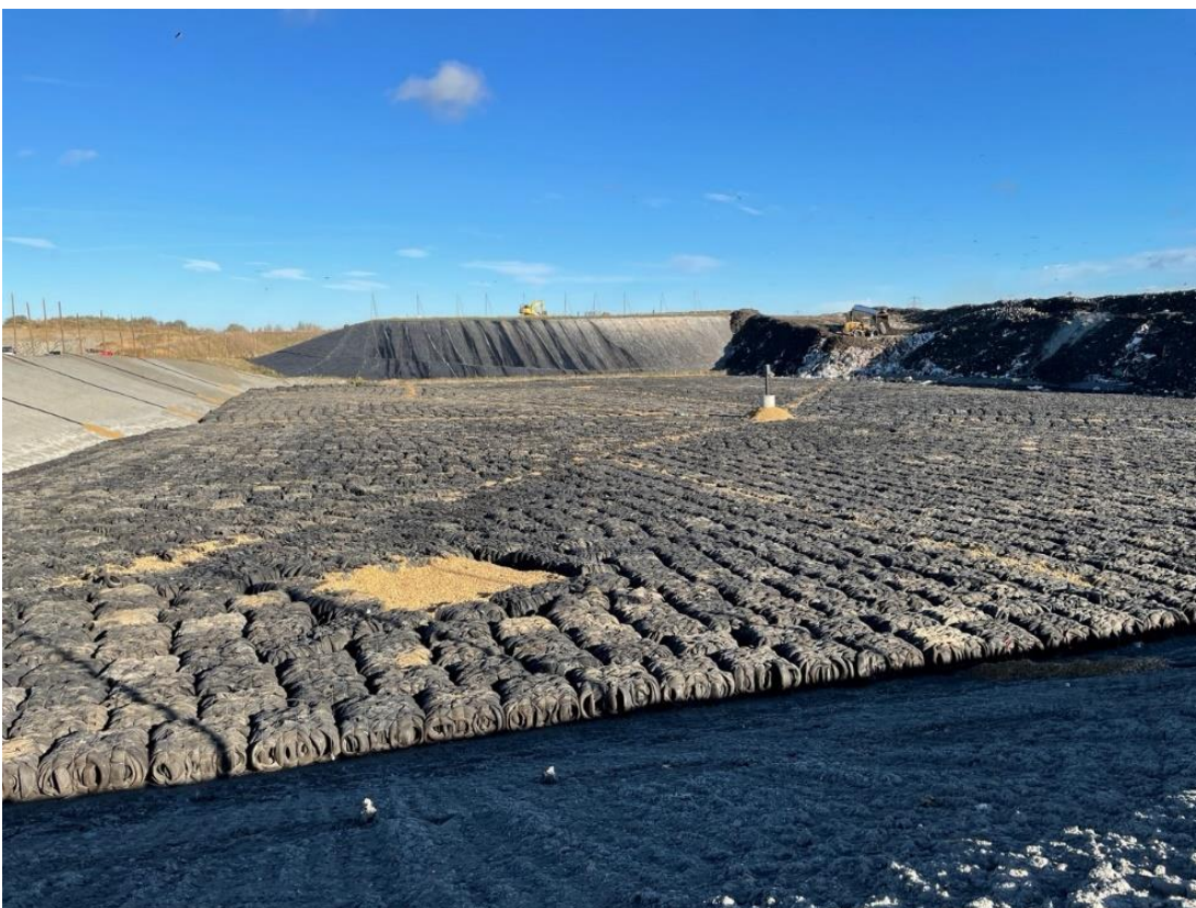
Figure NTS4: Eye Landfill, Southern Extension (Cell 4 prepared prior to landfilling, 2021)
