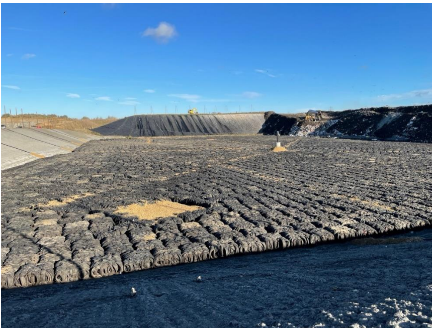
Figure 5: Southern Extension Area (Operational)
