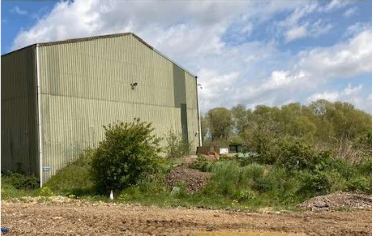
Figure PEA-7: Scattered Scrub within the Site
