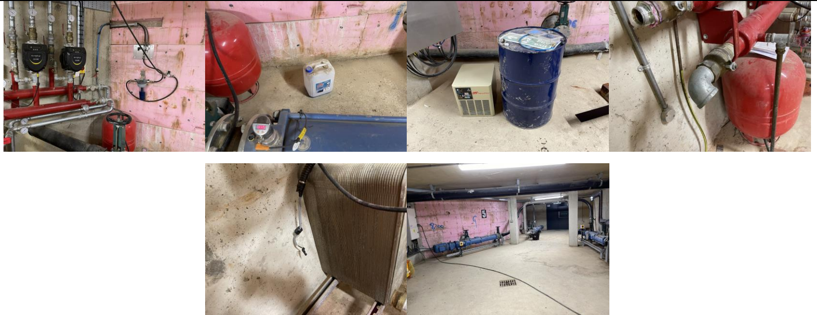
Housekeeping in Digester buildings
