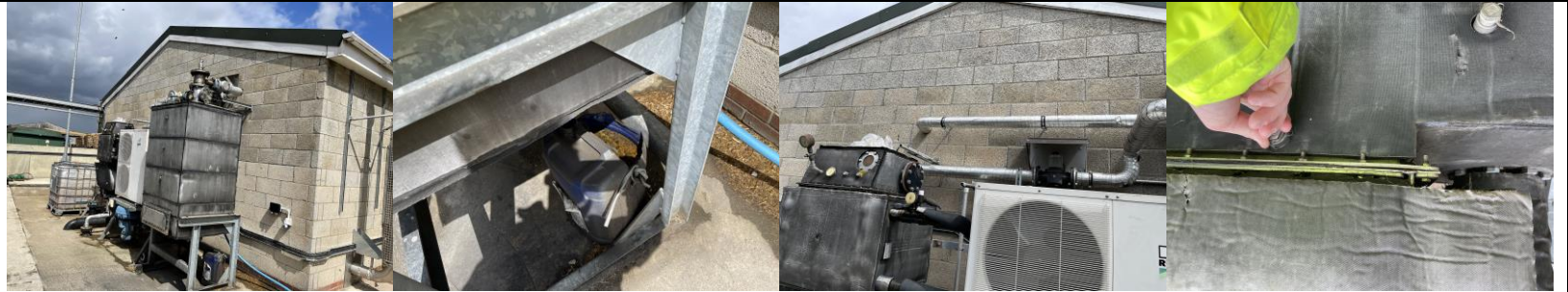
Gas Filter plant improvements
