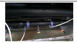
First, a coagulant, PAC, is added to **crack out the fats** and oils. The polluted matter is than destabilised and fine "floc" particles are formed.
