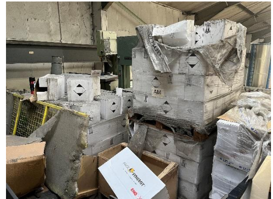
3 pallets of flammable products stored on mezz.
