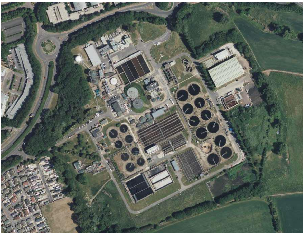
Figure 2-1- Satellite view of Oxford Sewage Treatment Works
