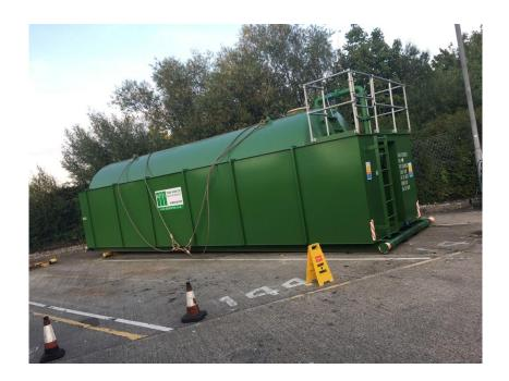
The manufacturer has confirmed that the tank and bund are designed to withstand the caustic nature of the wastewater. The bund is capable of holding 113.7% of the nominal contents of the tank and is therefore in line with Environment Agency guidance that it must be capable of holding a minimum of 110% of the capacity of the tank.
