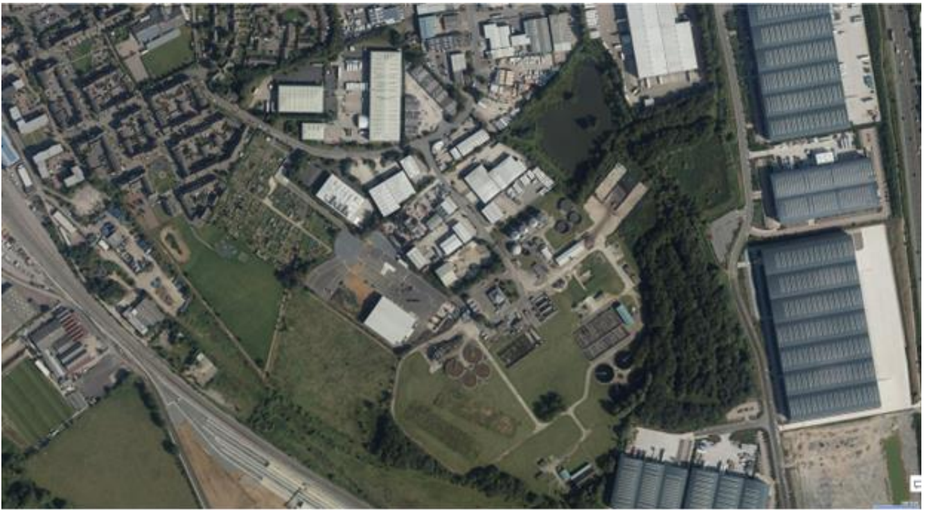
Figure 2-2 Satellite image of Banbury STW location next to industrial estate
