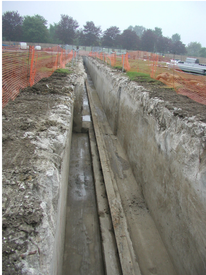
Figure 4.3. A view of the interior of Trench 2.
