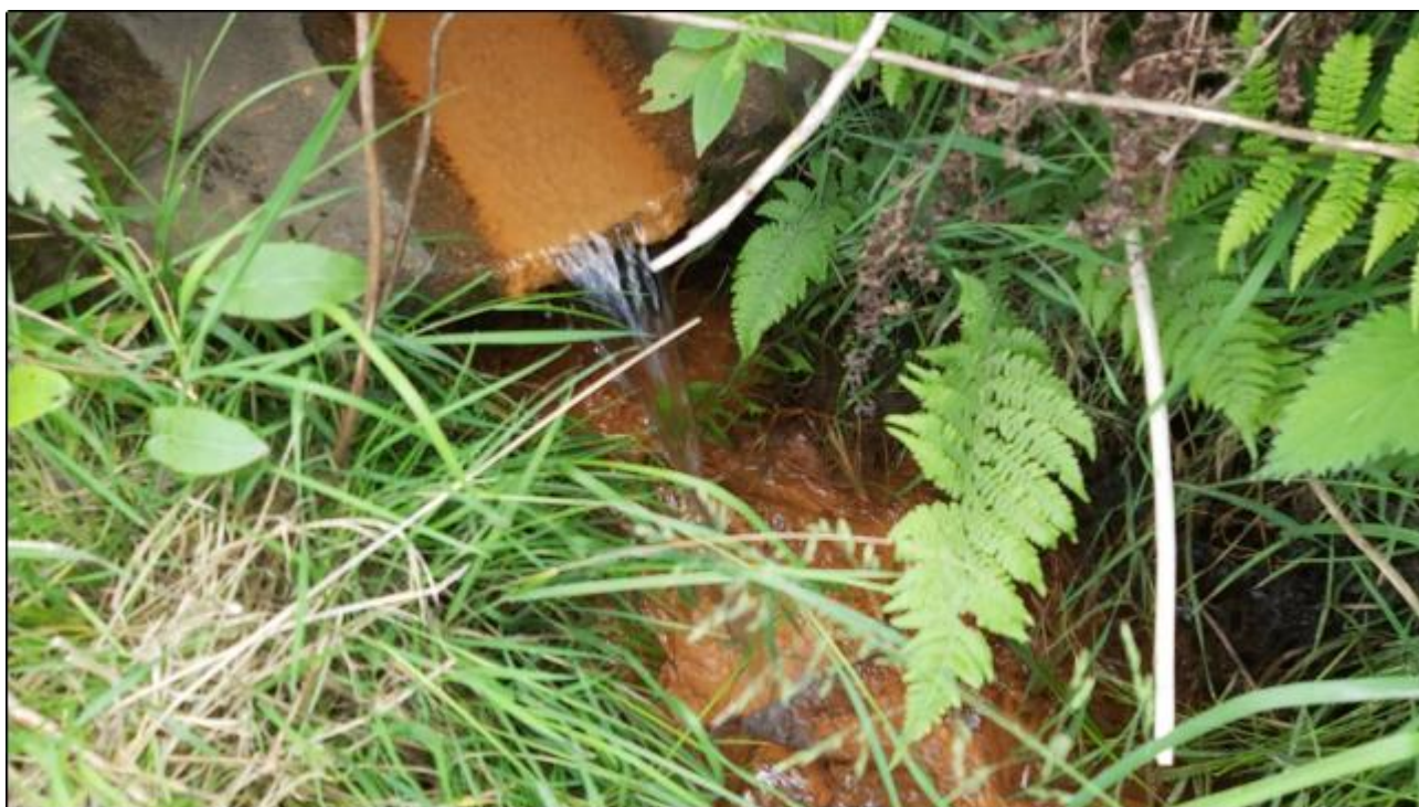
Mine Adit – measurement location west of end of adit where flow passes through a drainage pipe rather than in a ditch
