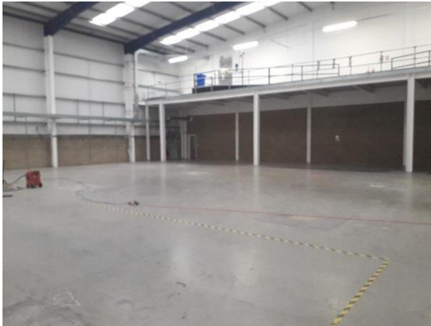
Photograph showing the internal layout of the eastern half of the building.
