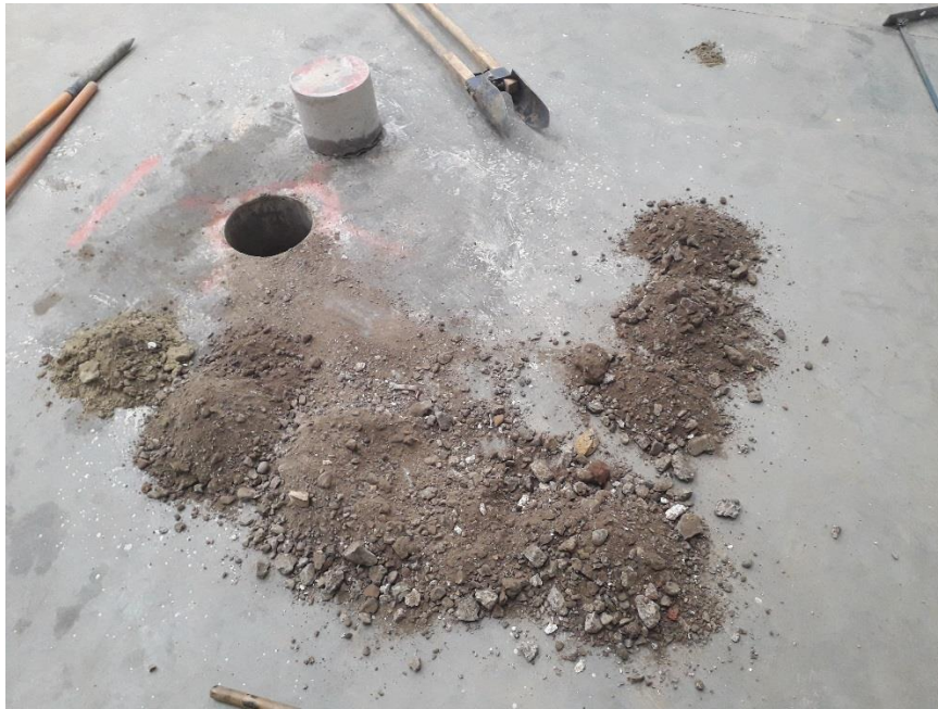
Photograph showing the nature of the concrete cores, sub-base and underlying Made Ground.
