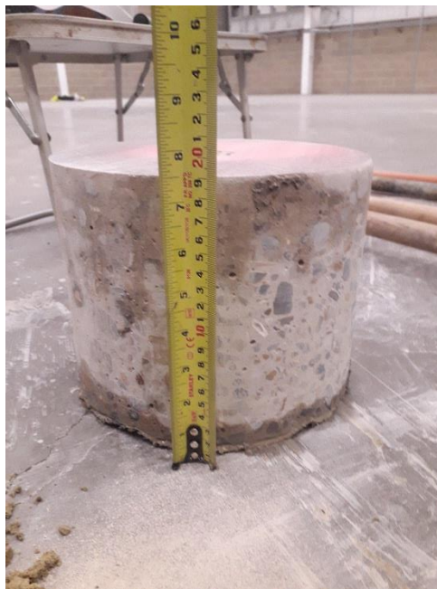
Photograph showing the concrete core in CC02.
