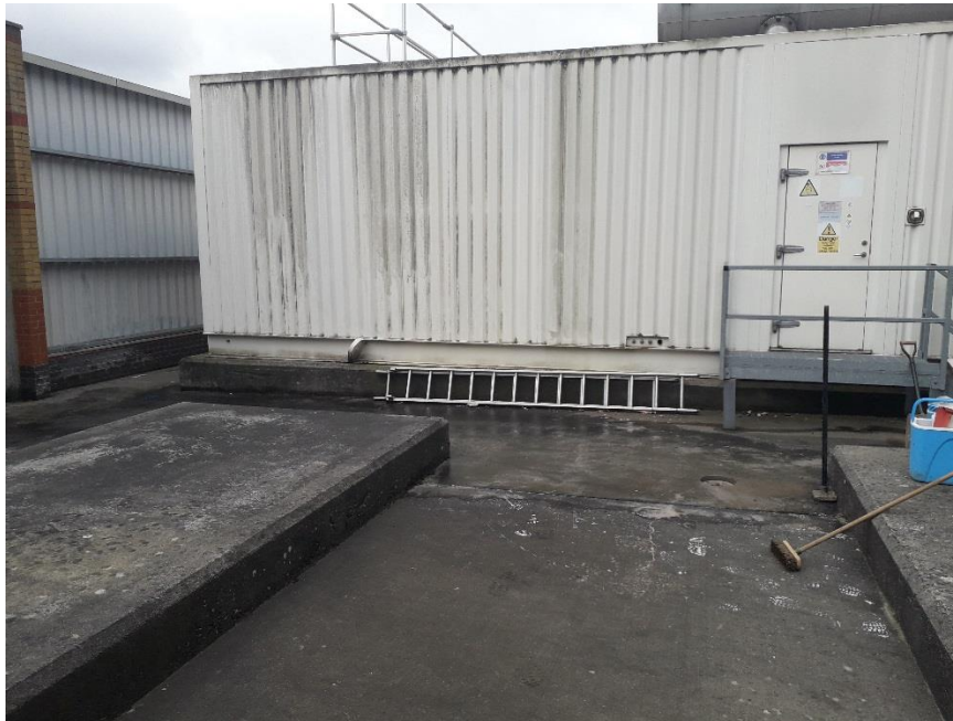
Photograph showing the location of CC07 and the external slabs.
