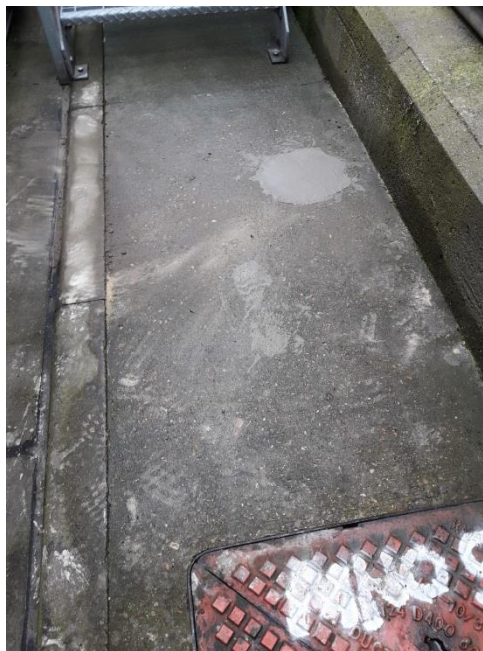
Photograph showing the location of CC06, post reinstatement.
