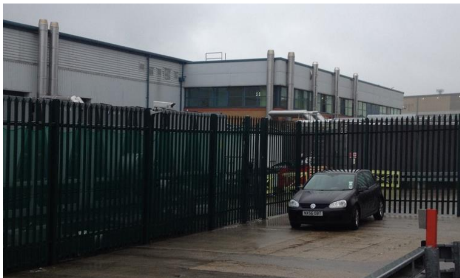
Figure 3.2 – Existing Generator Flues
