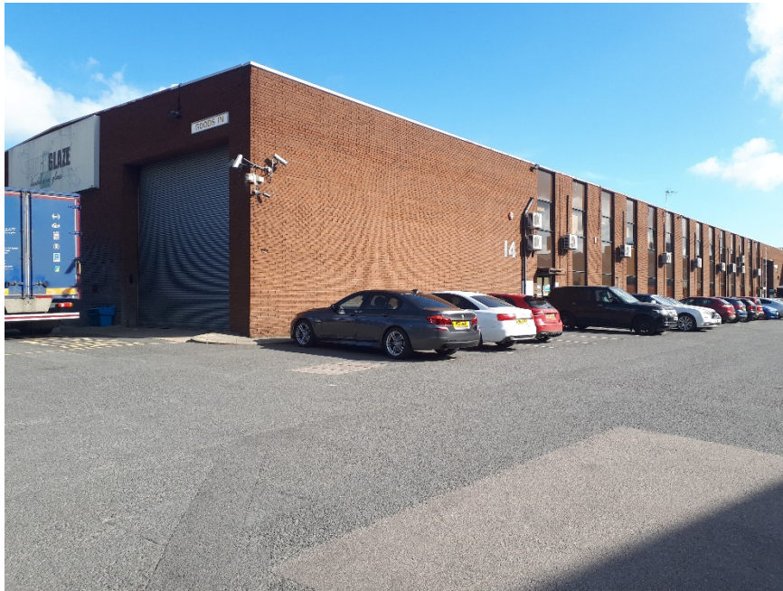
Photo 3. View of Unit 14 from the site entrance.
