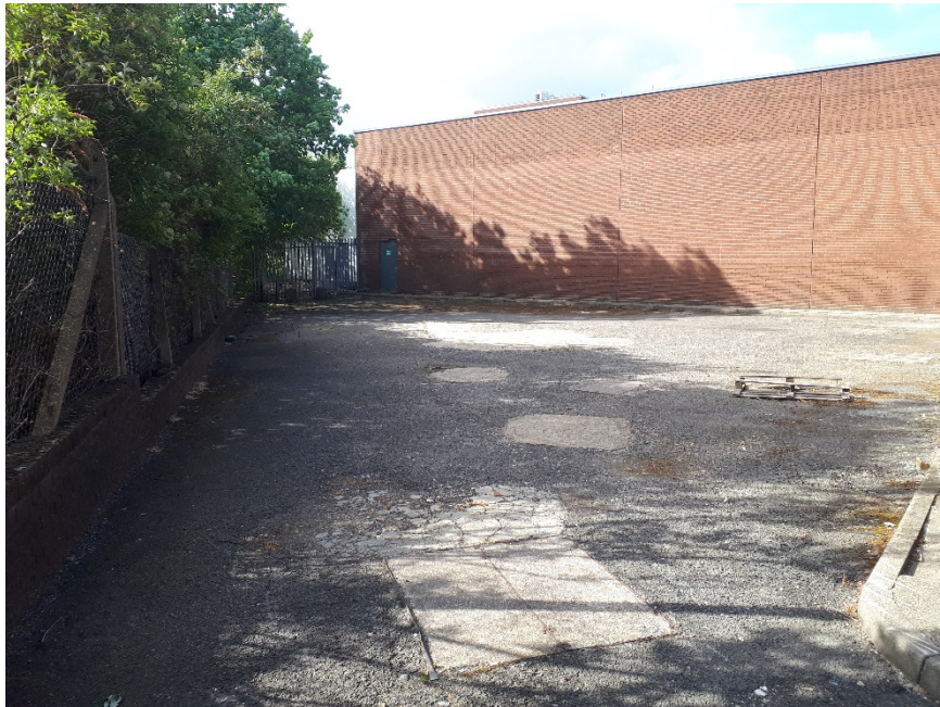
Photo 8. Triangular parcel of land in the south-east of the site (Plot 175a).
