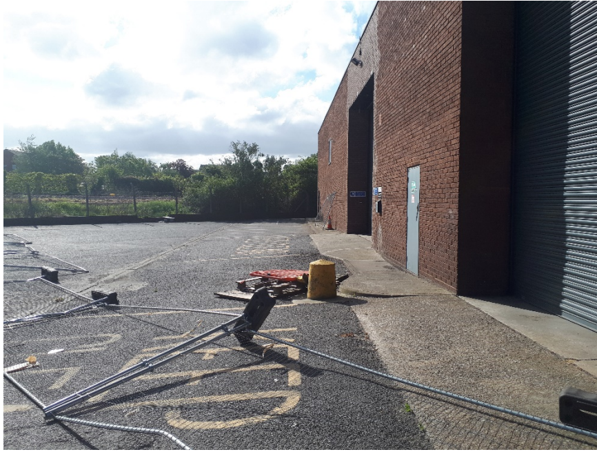
Photo 7. Service yard to the east of Unit 8.
