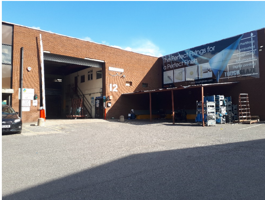
Photo 5. View of Unit 12 from the centre of the site, looking north.
