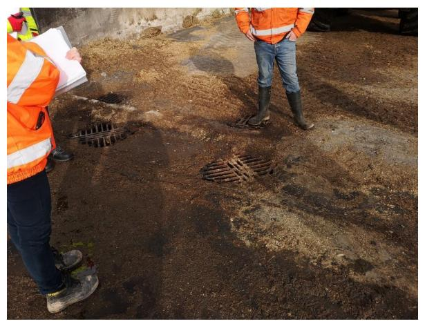
Photograph 4: Existing silage clamp drains
