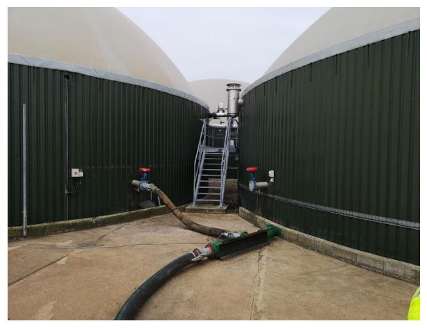
Photograph 14: Existing digesters with concrete surround, gantry and pressure relief valve
