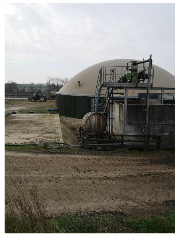
Photograph 10: Existing digestate separator, buffer tank and fibre concrete storage bay
