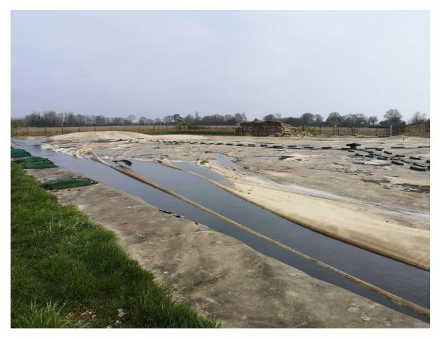
Photograph 6: Existing covered digestate storage lagoon with straw stored in the background. Maintenance and repair of the cover is being undertaken.
