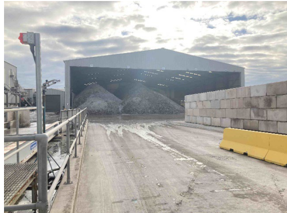
View of IBA reception shed
