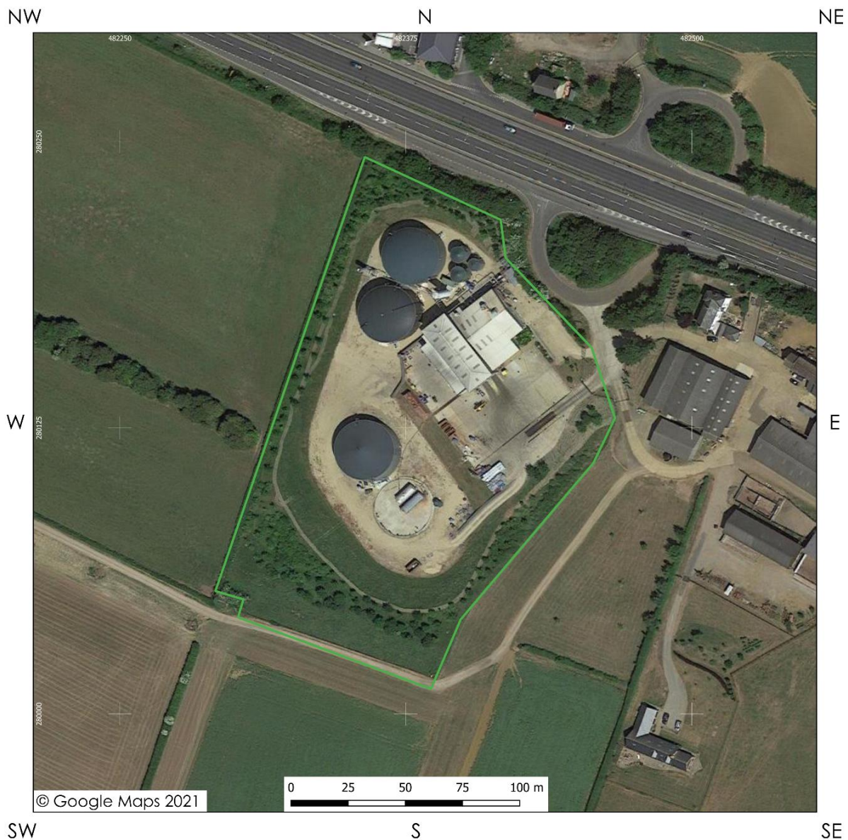
Figure 1. Aerial image of site
