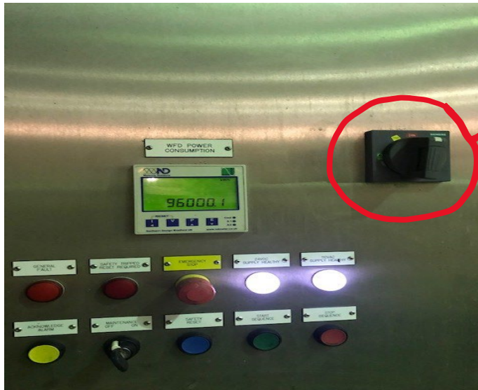
Secondary isolation – local isolation number: MOTOR RF101
