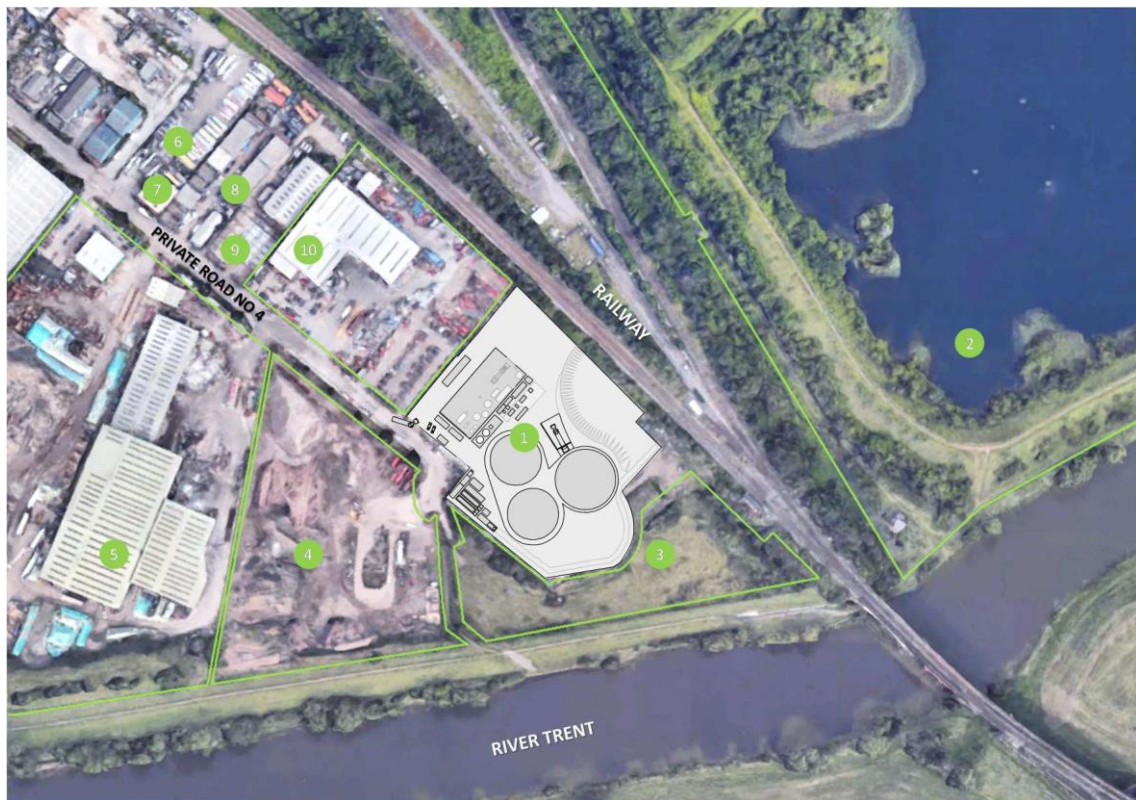
Figure 1 Site location: The Colwick AD facility and neighbouring premises. (1) Bio Dynamic (UK) AD Facility, (2) Netherfield Lagoons, (3) Canal & River Trust, (4) Merlin Environmental Ltd, (5) Enva England Ltd, (6) Tiger European (UK) Ltd, (7) Aggregate Industries UK Ltd, (8) NG4 Car Services Mechanik Nottingham, (9) Nottingham Powdercoating Ltd, (10) Enva England Ltd
