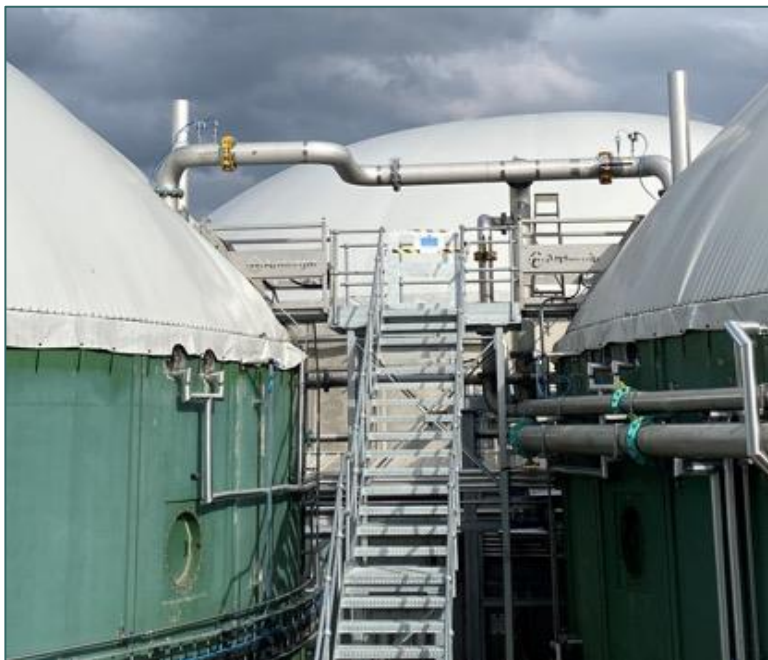
Image 3: Gas Storage Roofs and Gantry
