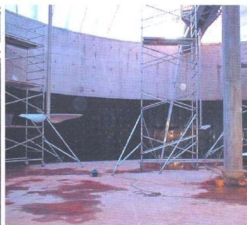
Storage tank retrofitted with a bolted-on thermoplastic lining – Bolted Lining™ System.
