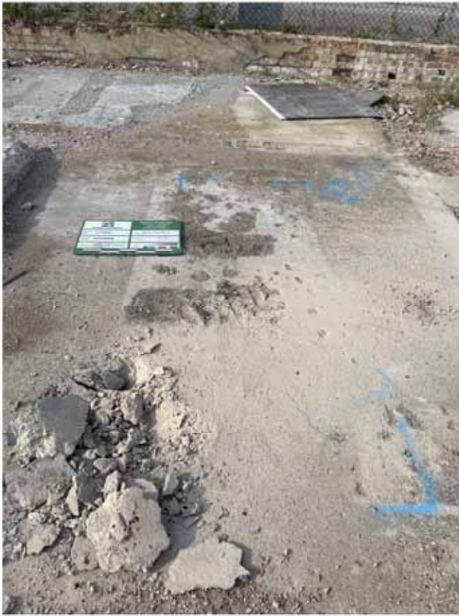
1. Prior to excavation
