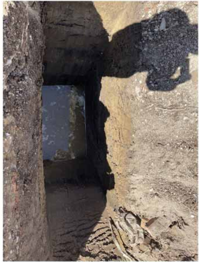
6. Base and groundwater
