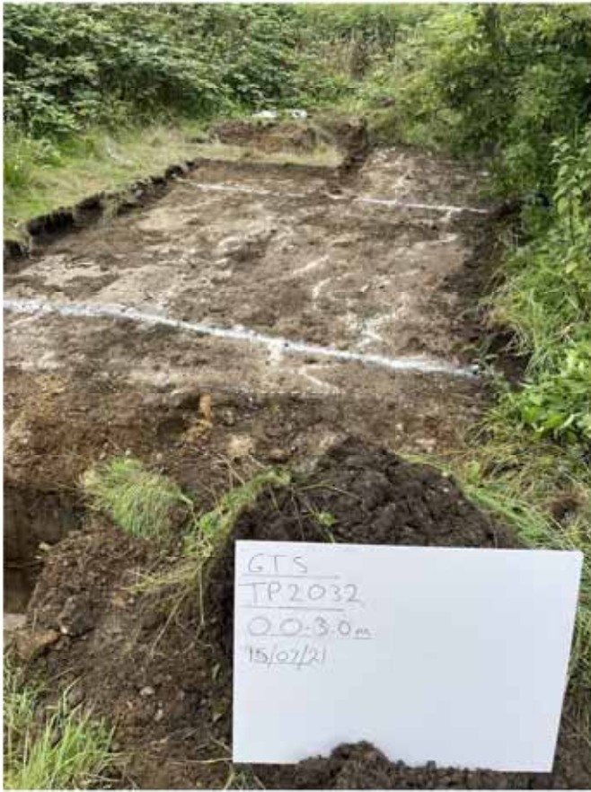
1. Location and shallow excavation
