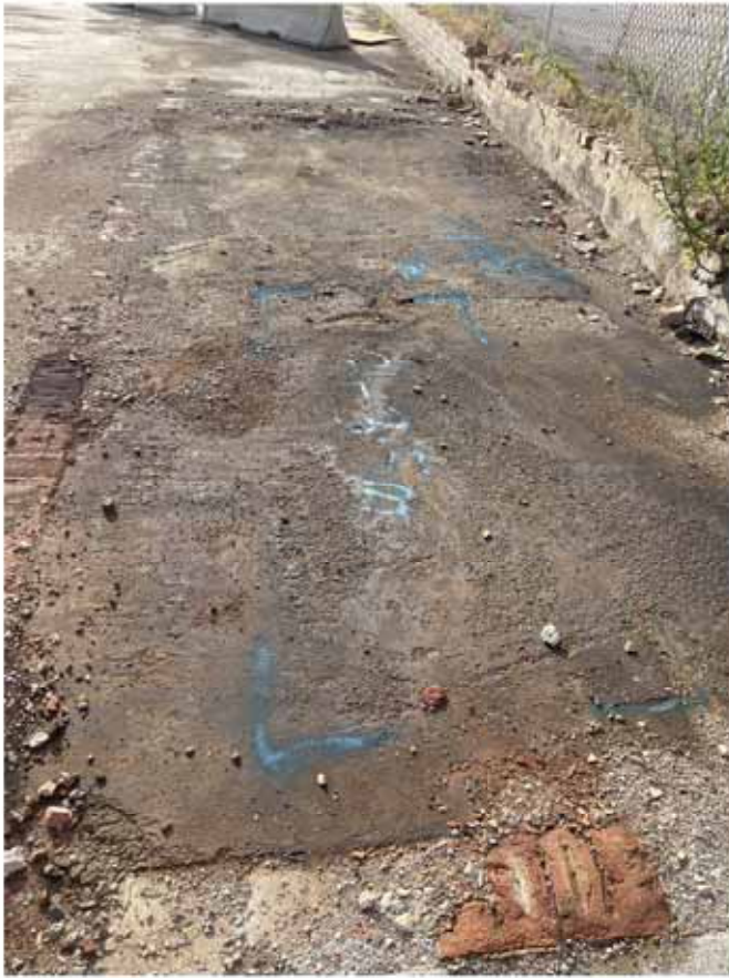
1. Prior to excavation
