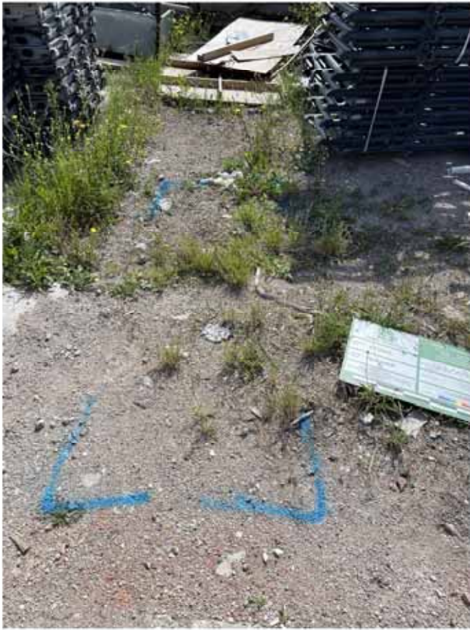
1. Prior to excavation
