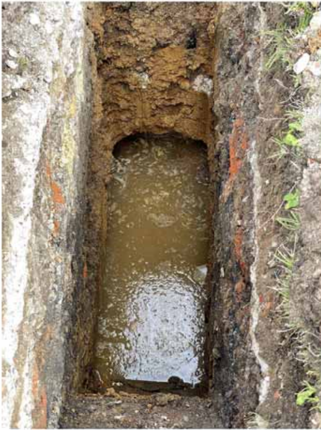
5. Base and groundwater
