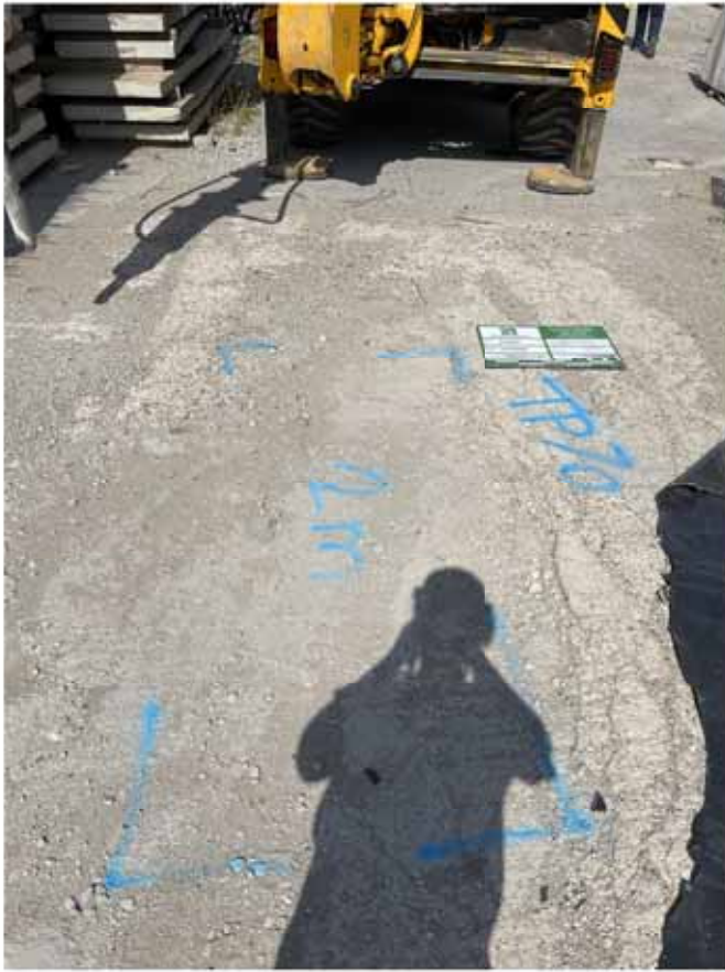
1. Prior to excavation
