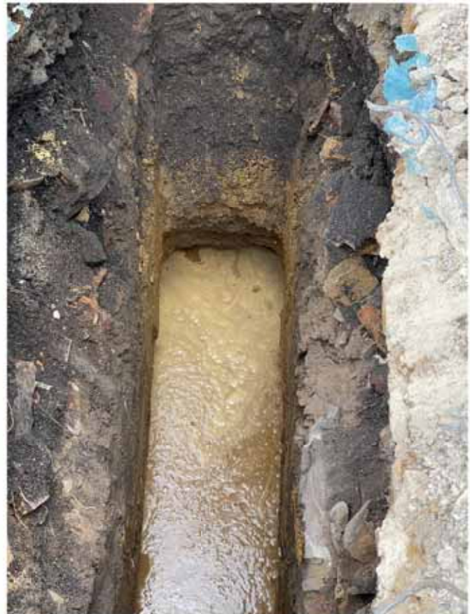
4. Base and groundwater
