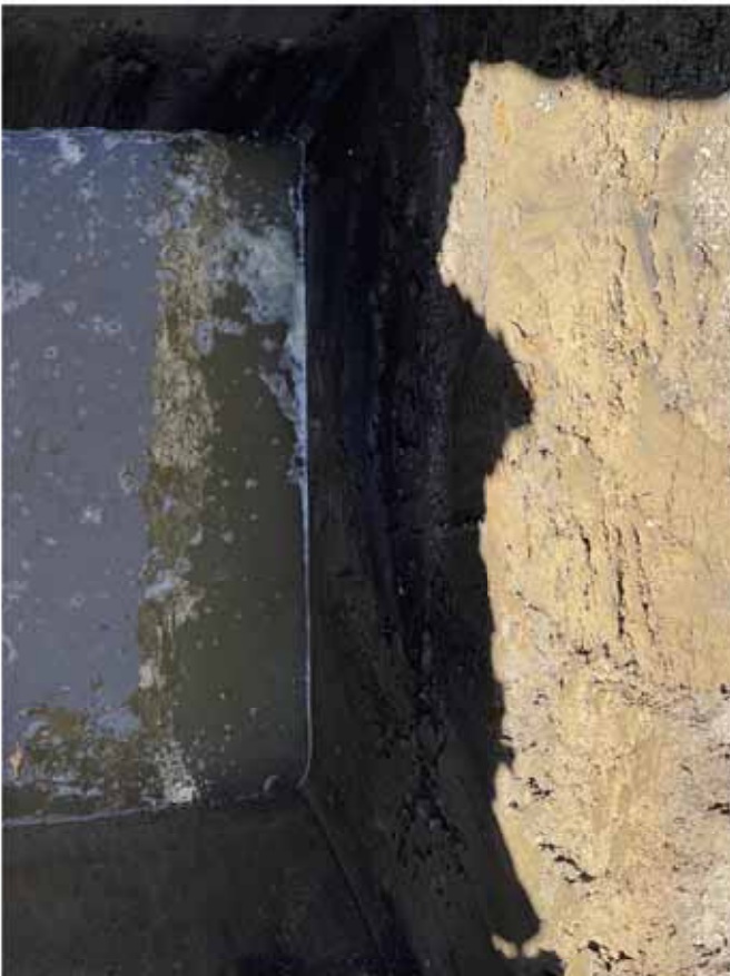
7. Side and base with groundwater
