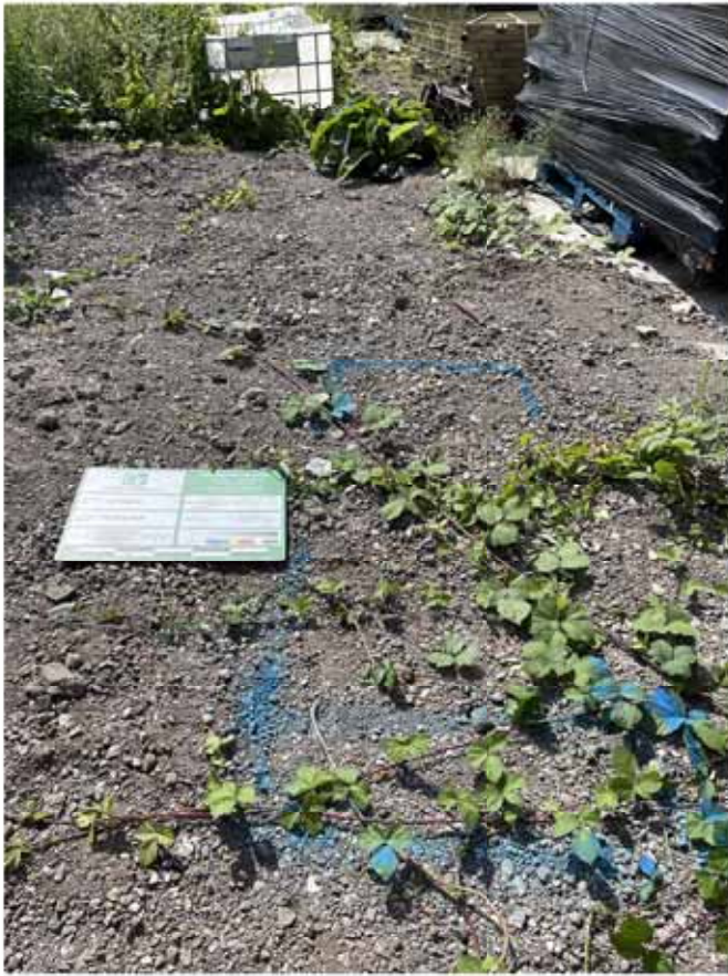
1. Prior to excavation
