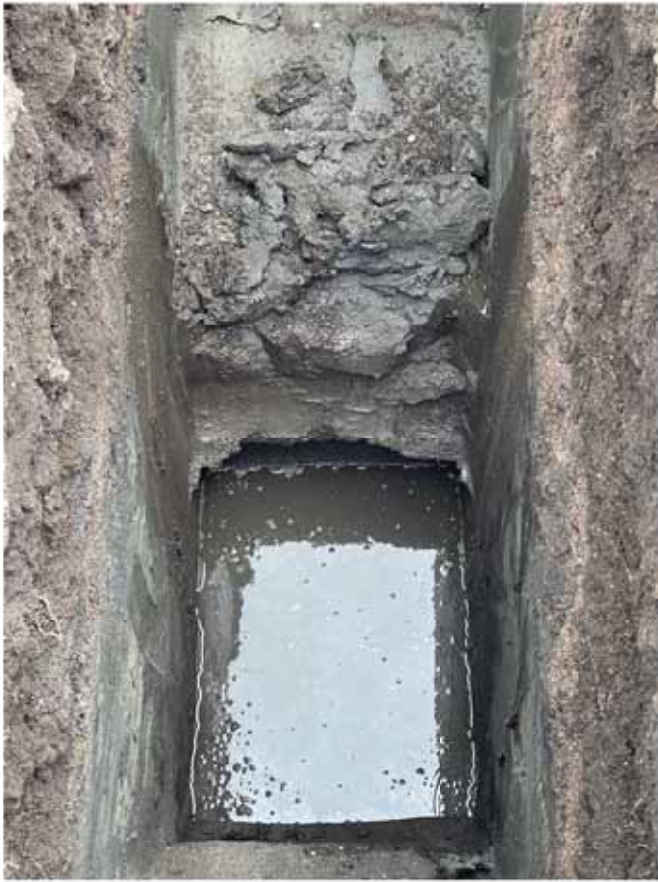
5. Base and groundwater
