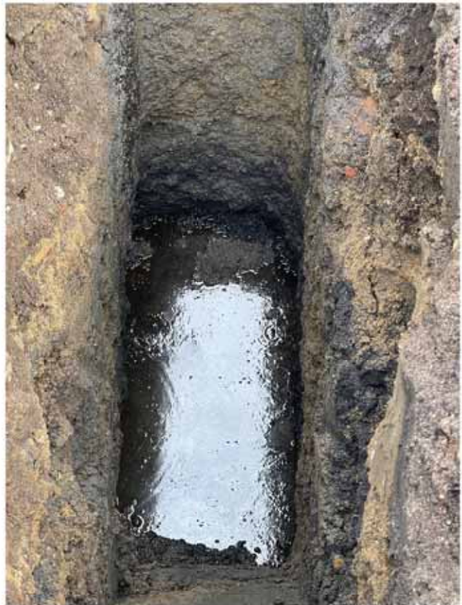
4. Base and groundwater
