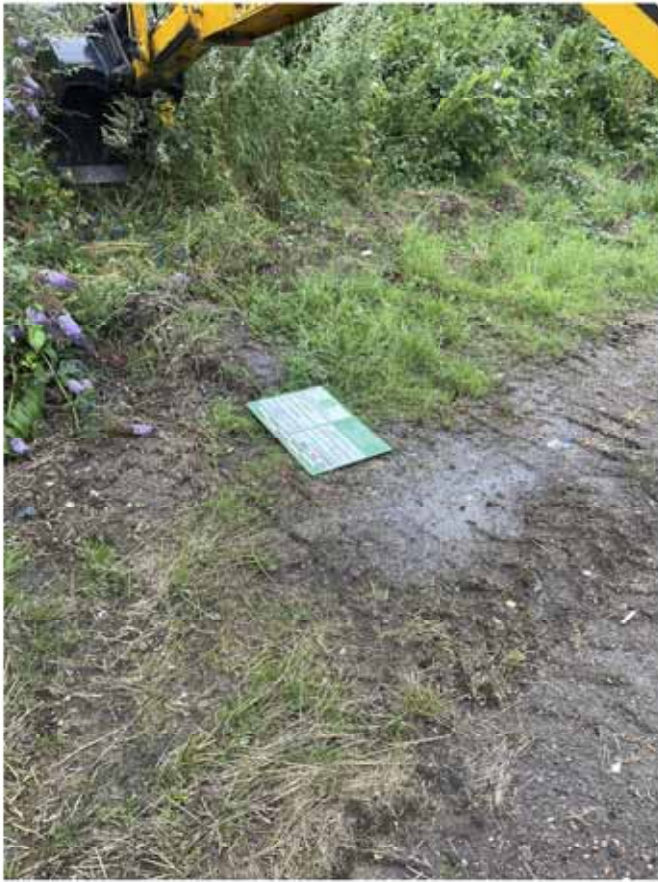
1. Prior to excavation
