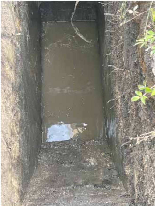
3. Base and groundwater
