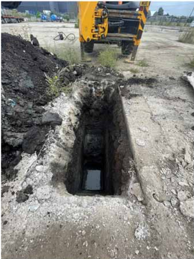
3. Excavation and spoil
