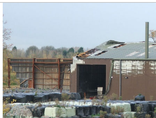
Photograph 6. The Minerals Recycling Facility (TN10).
