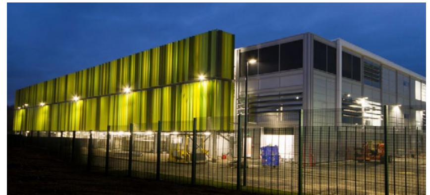
Example of articulating facade elements to create a striking Data Centre
