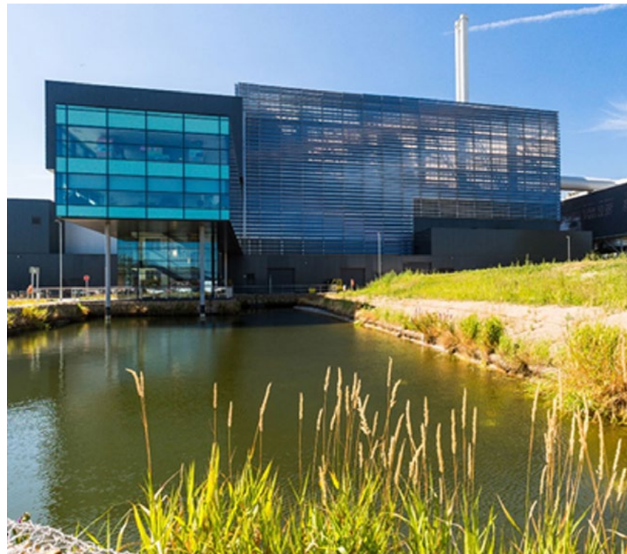
Suffolk Energy from Waste Plant
