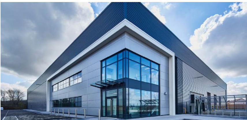
Office Element Acting as a Landmark Feature
