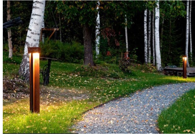
Low level lighting
