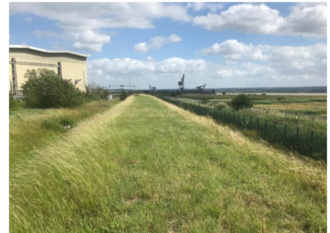
Flood defence bund on the western Site boundary screens the Site (left) from the Hoo Marshes (right)
