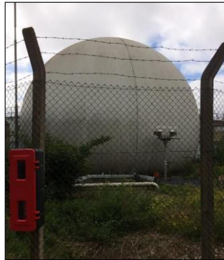
Figure 8: Double membrane gas holder.
