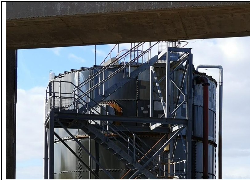
Fixing of tank - patches
