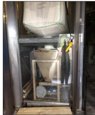
Figure 6: Polyelectrolyte dispenser.
