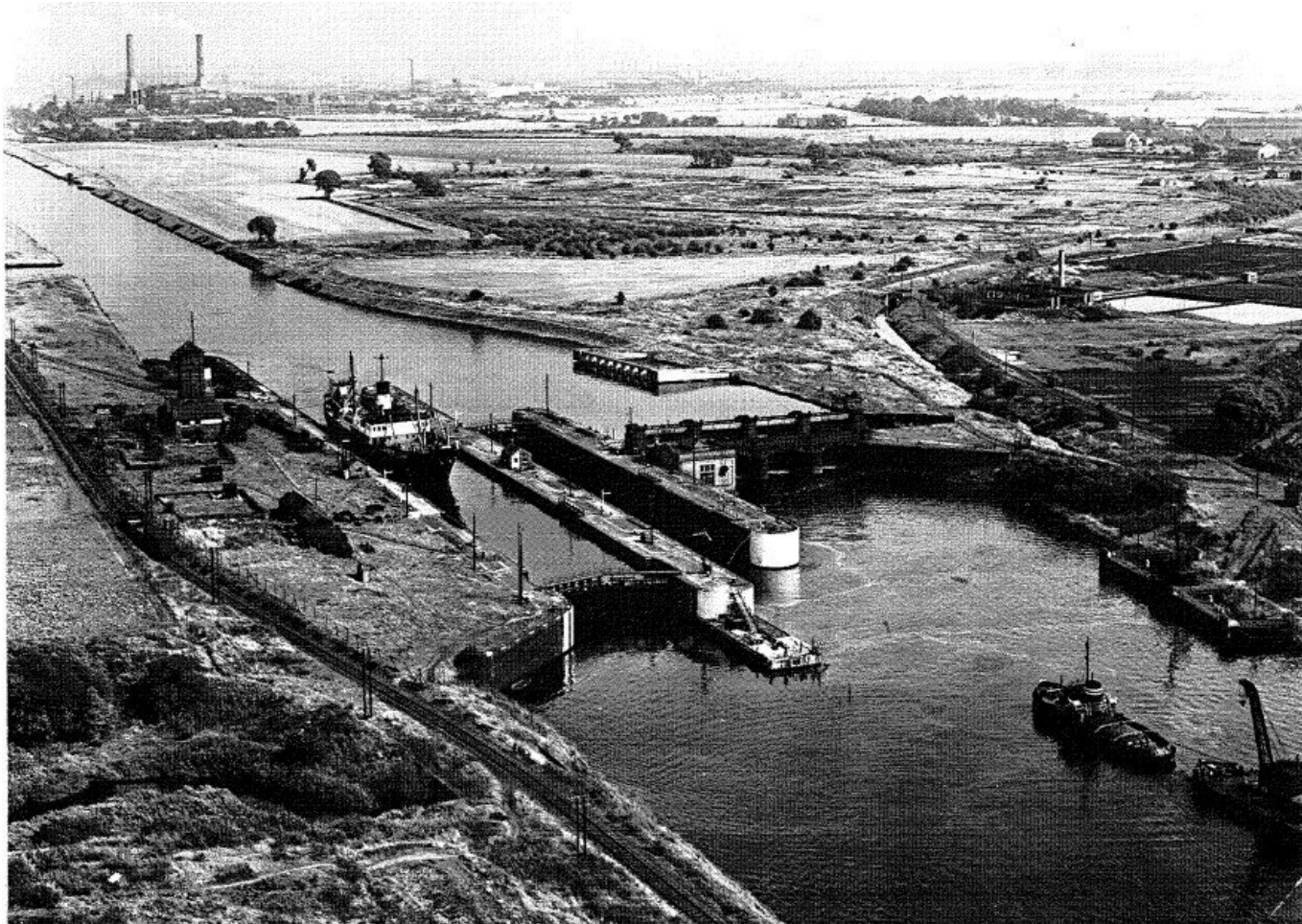
Plate 6: Historical aerial view of Barton Locks looking eastwards. Date of photograph unknown but believed to be circa 1930's. Note the tram-ways which extended across the length of the Port Salford berthing area
