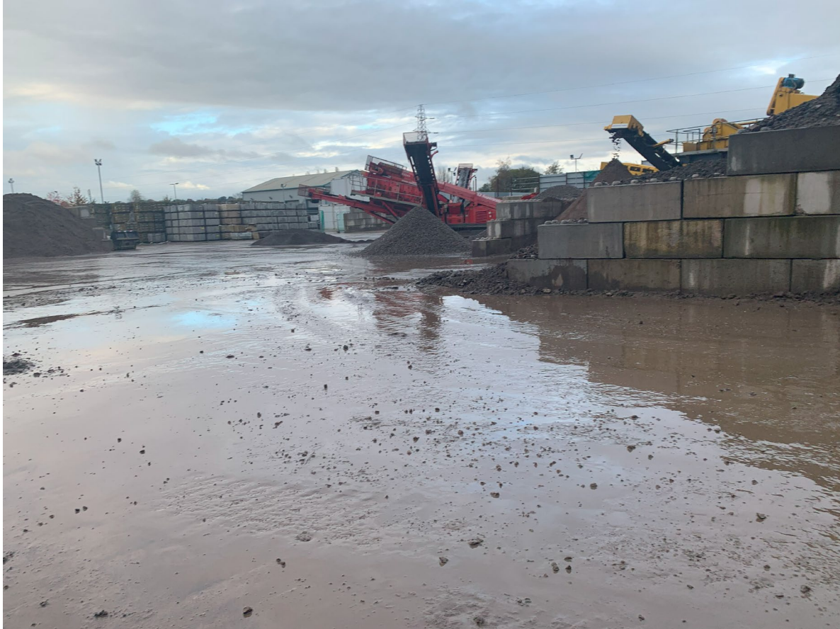
Photo 3: Temporary wash plant under trial
