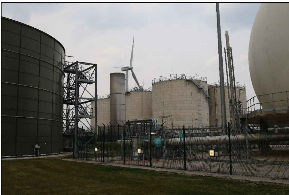
Figure 14. Dewatering feed tank (green tank to the left).
