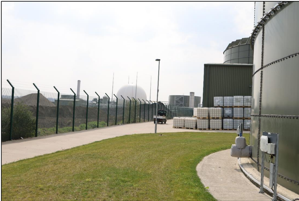
Figure 11. Sludge thickener feed tank (first on the right).
