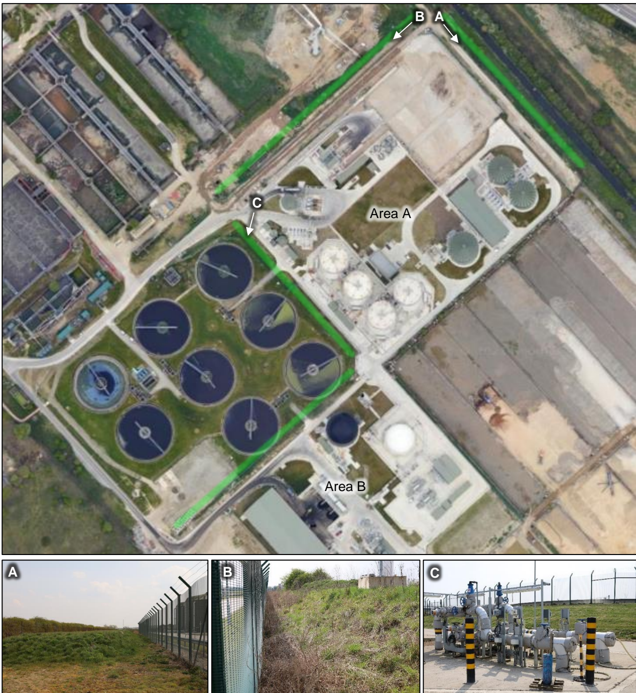
Figure 29. Existing areas of raised ground situated between Areas A and B, and the Wyke Beck and WwTW.
