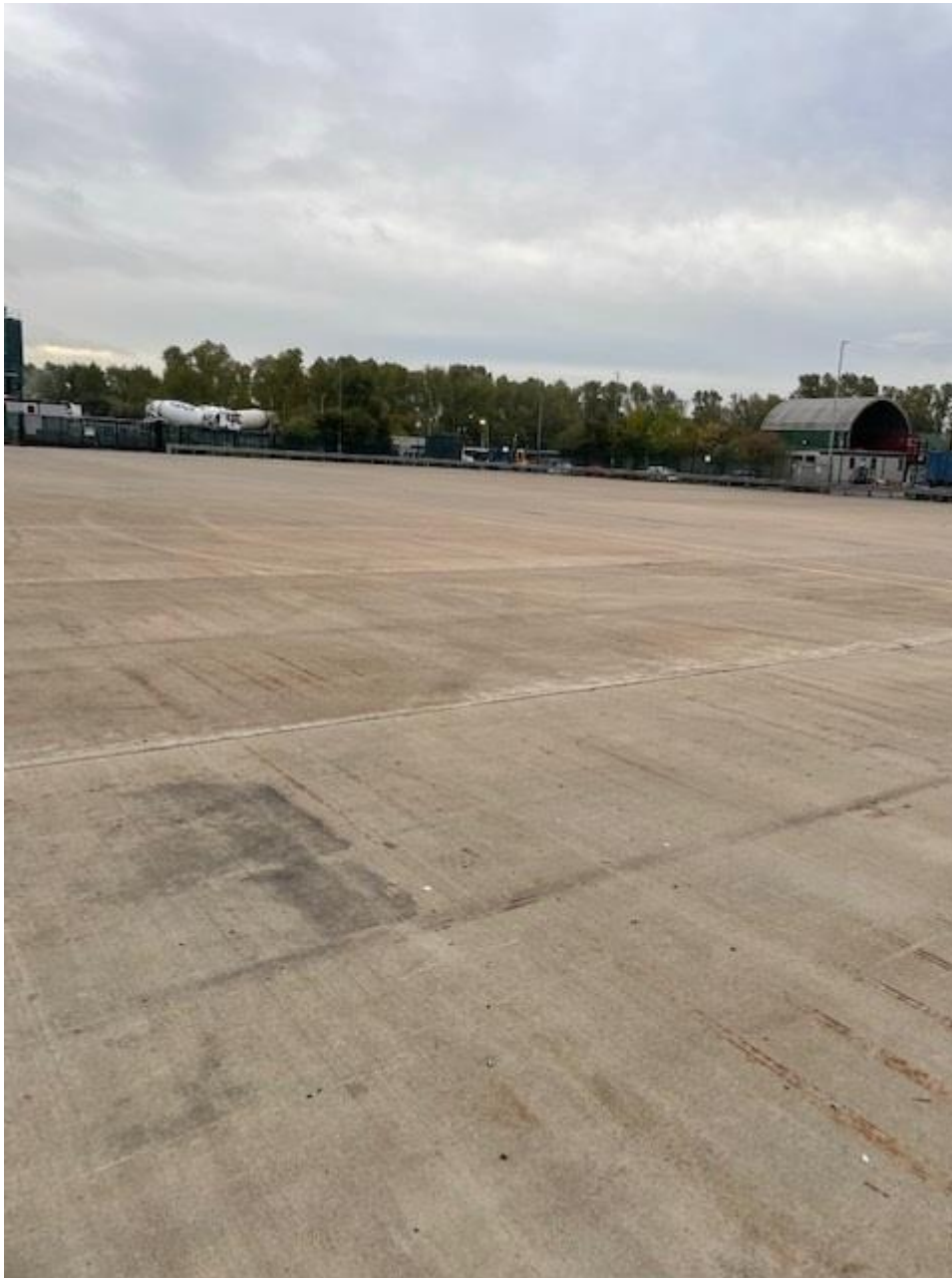
Storage yard and acceptance area – site surfacing
