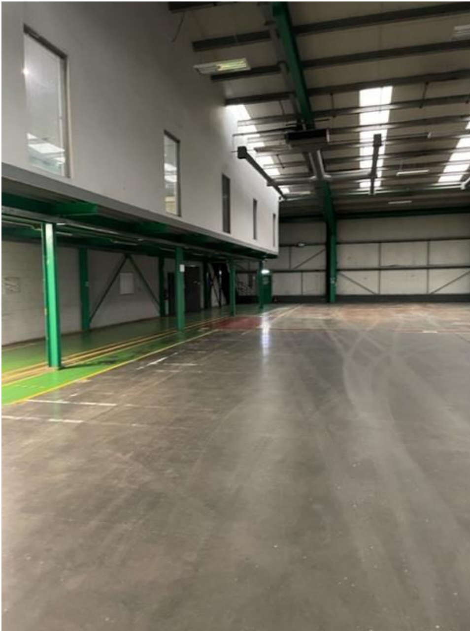
Inside storage shed – surfacing and infrastructure
