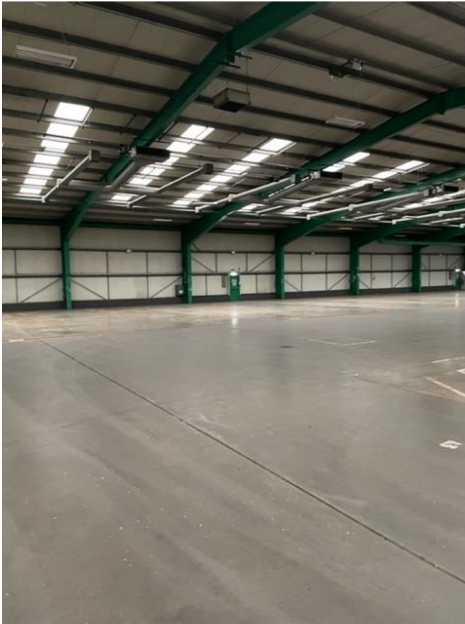
Inside storage shed – surfacing and infrastructure
