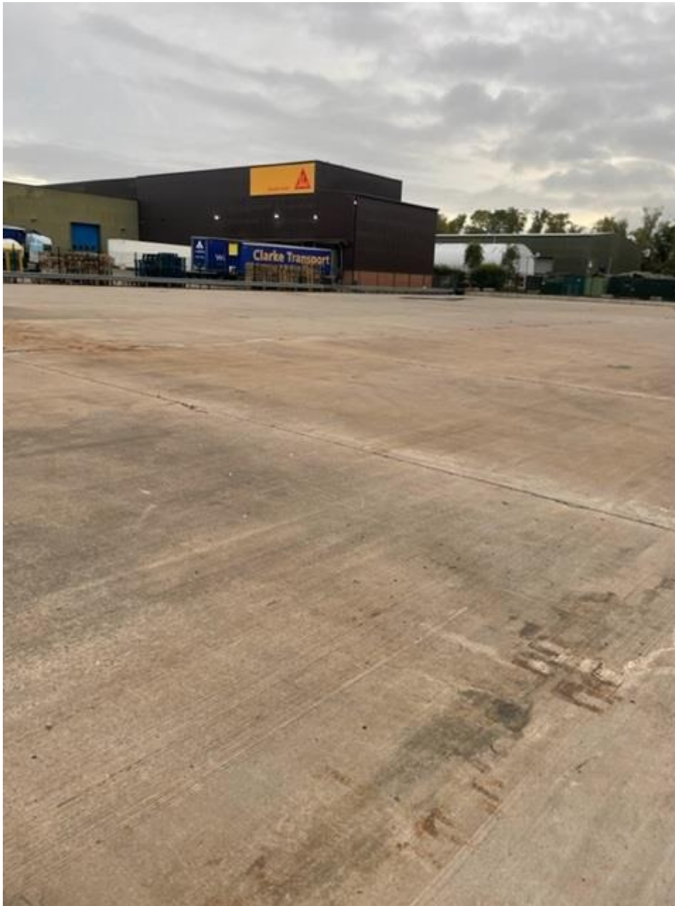
Storage yard and acceptance area – northern boundary
