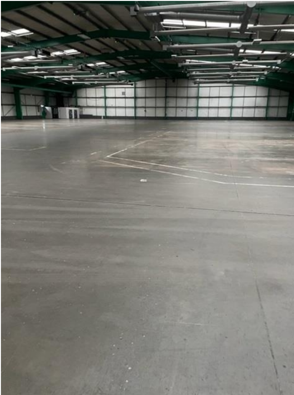
Inside storage shed – surfacing and infrastructure
