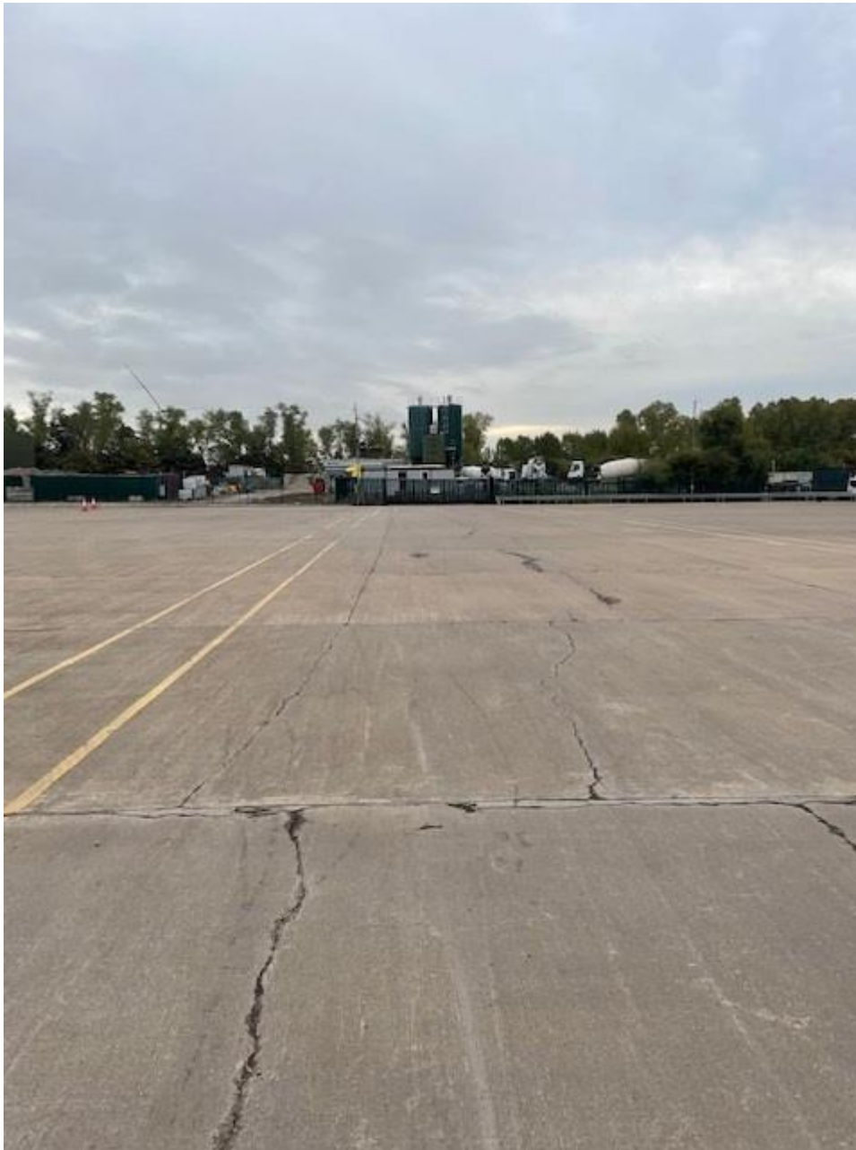
Storage yard and acceptance area
