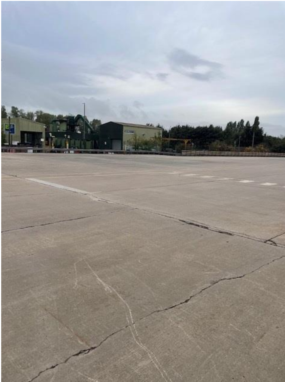
Storage yard and acceptance area
