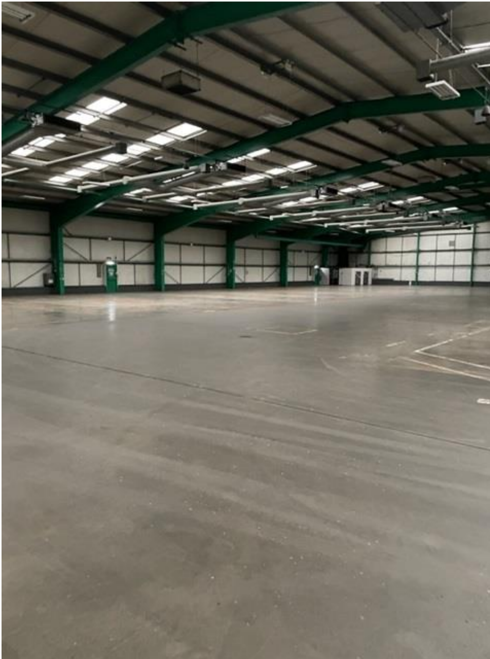
Inside storage shed – surfacing and infrastructure
