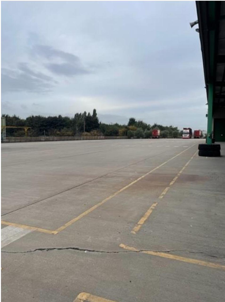
External yard area adjacent to warehouse/storage building
