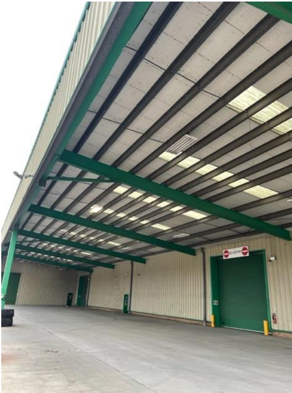
Canopy to warehouse/storage building
