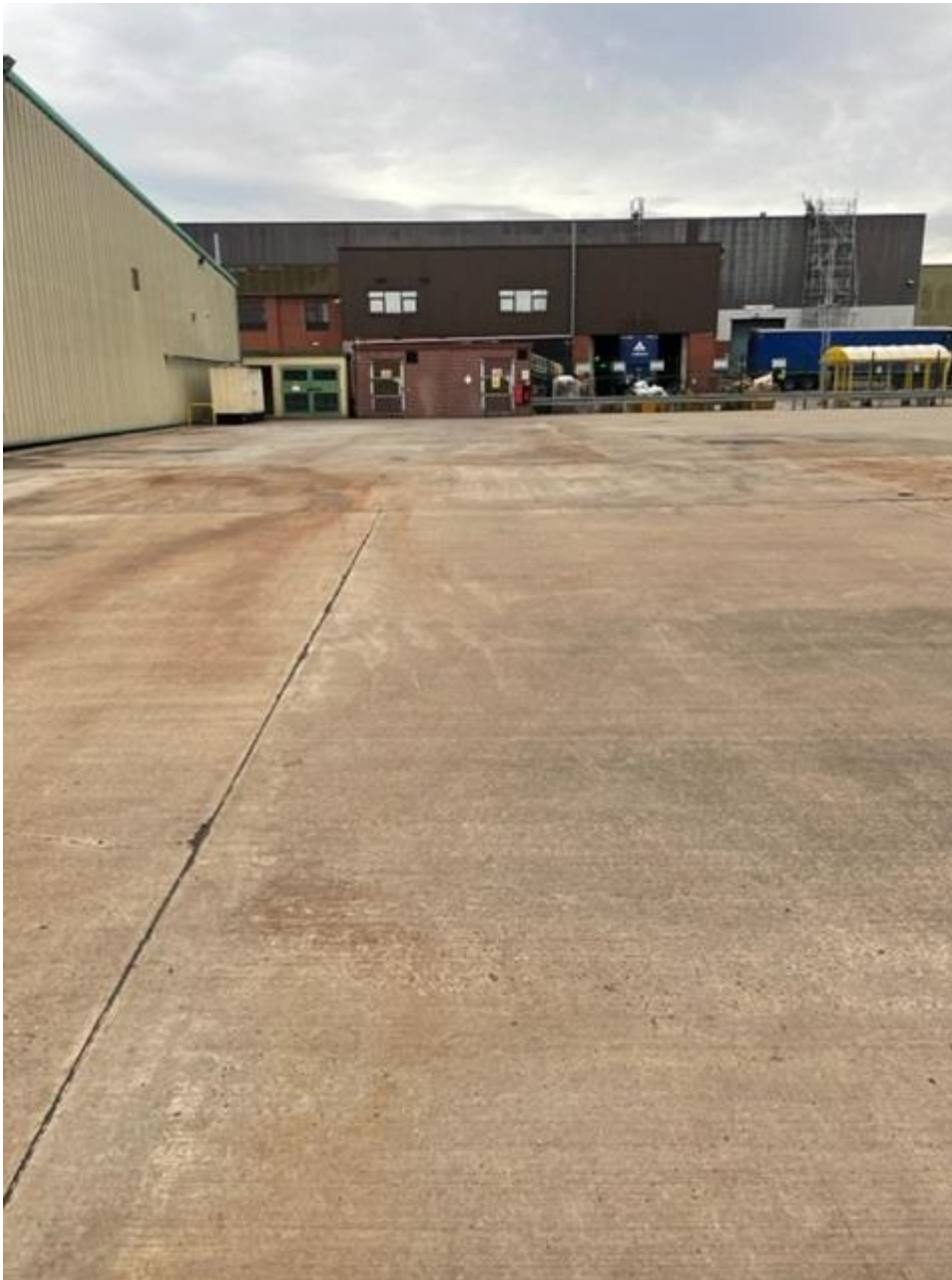
Storage yard and acceptance area – northern boundary
