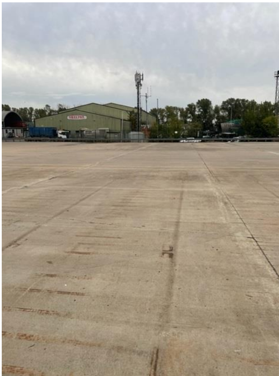
Storage yard and acceptance area
