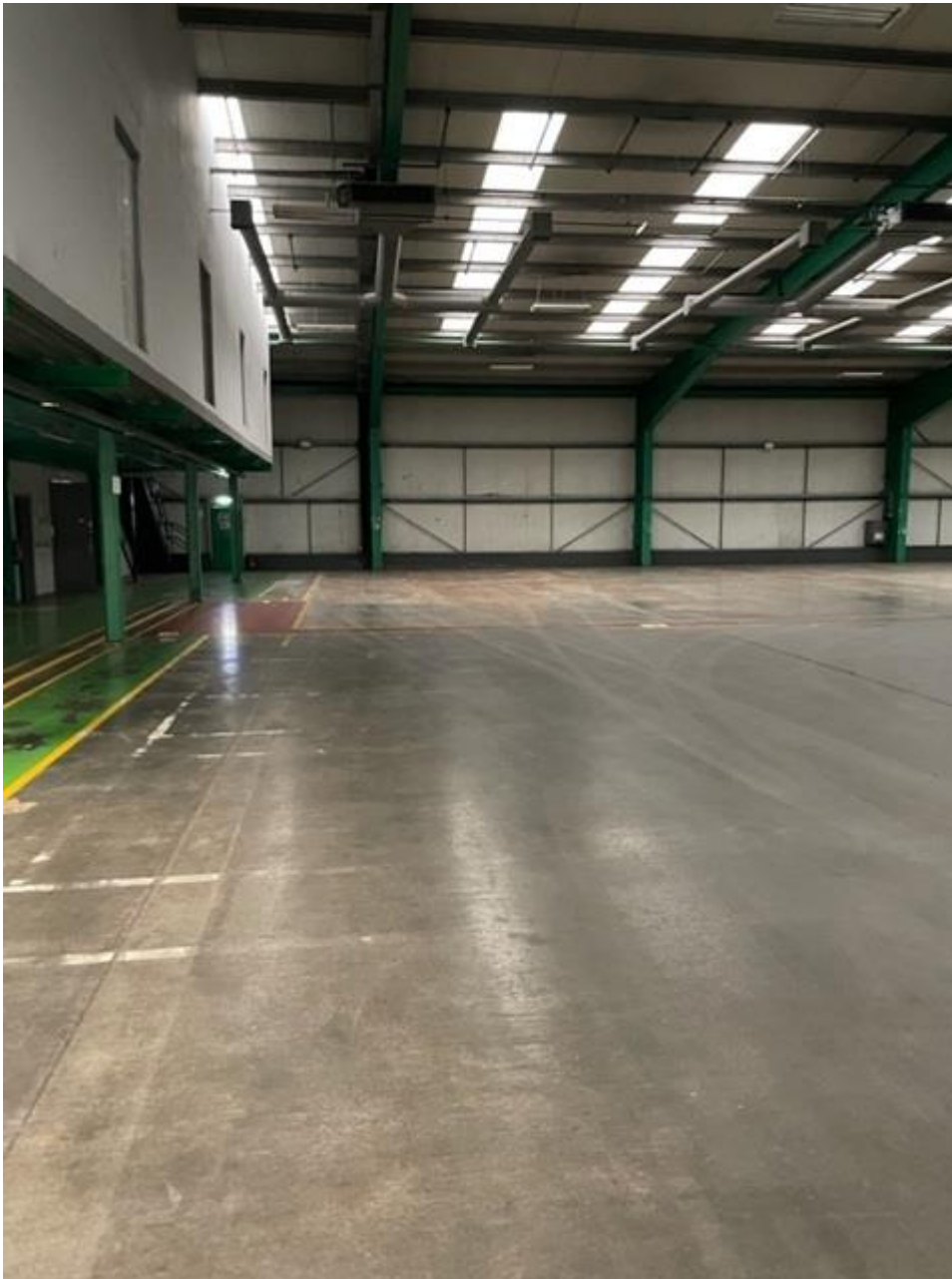
Inside storage shed – surfacing and infrastructure
