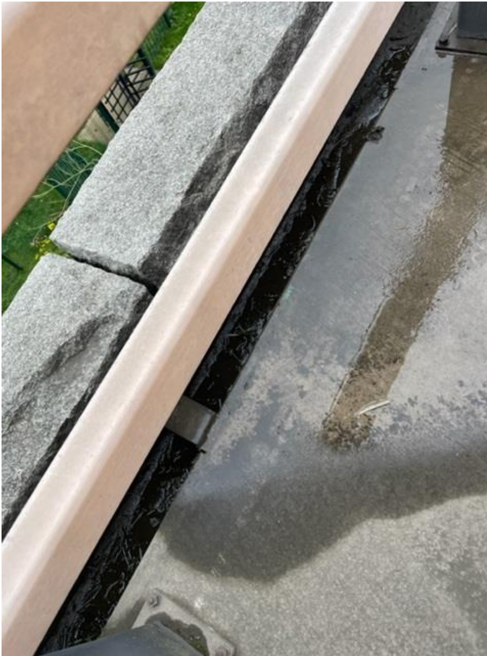
Drainage Channel – southern boundary
