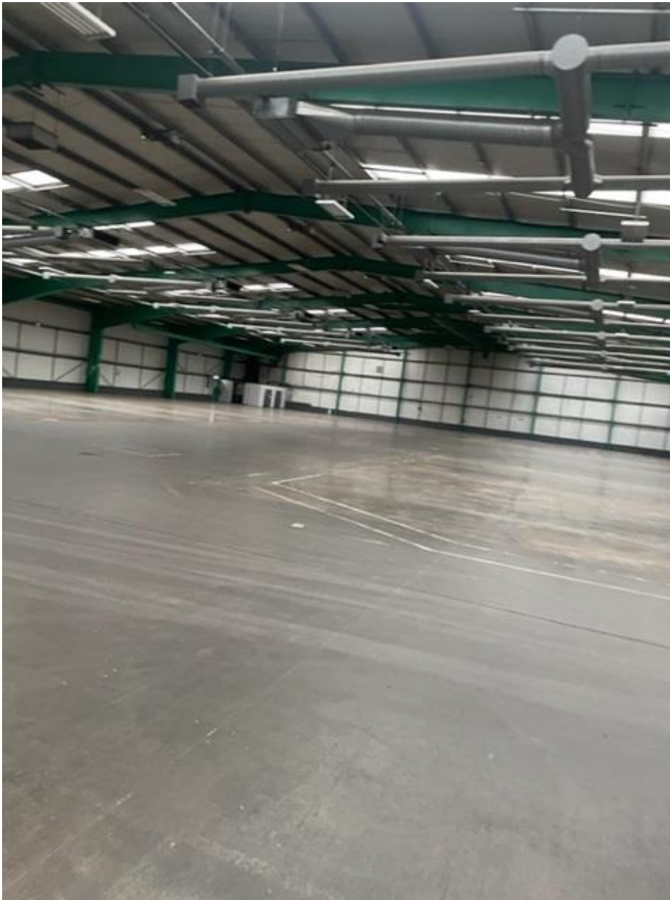
Warehouse – proposed treated wood storage area
