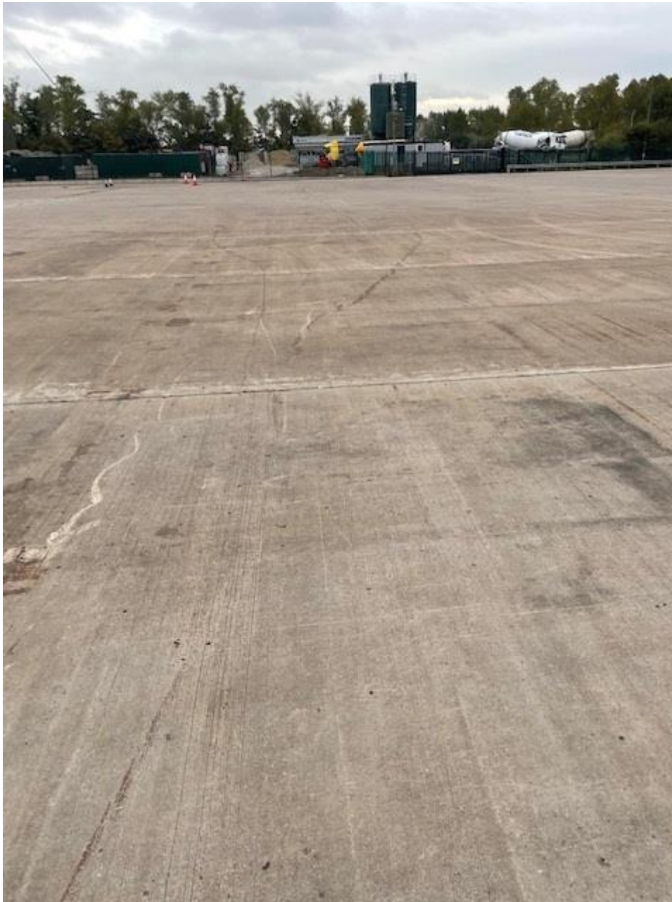
Storage yard and acceptance area – surfacing
