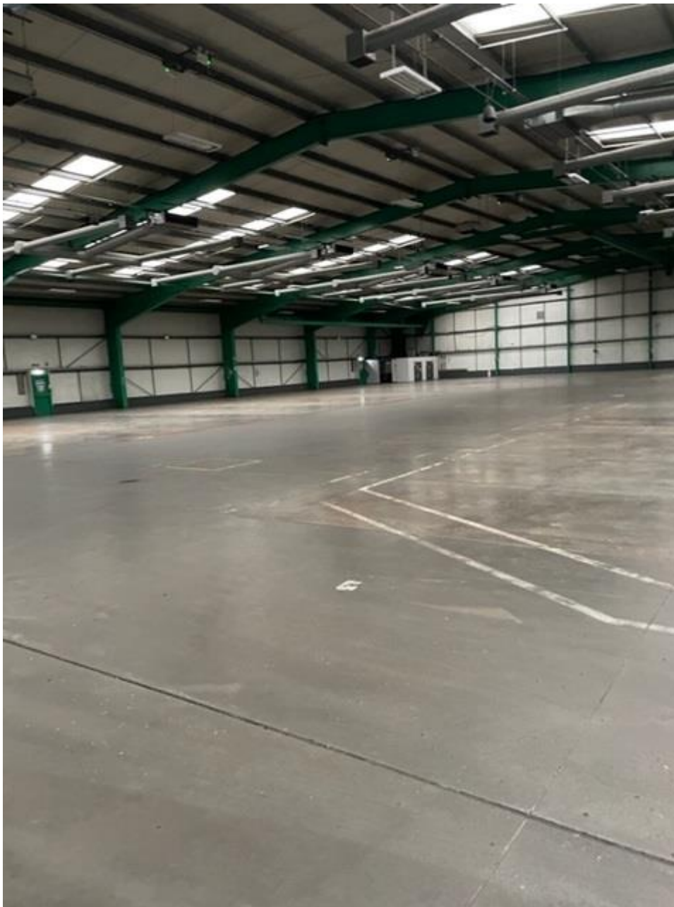
Inside storage shed – surfacing and infrastructure
