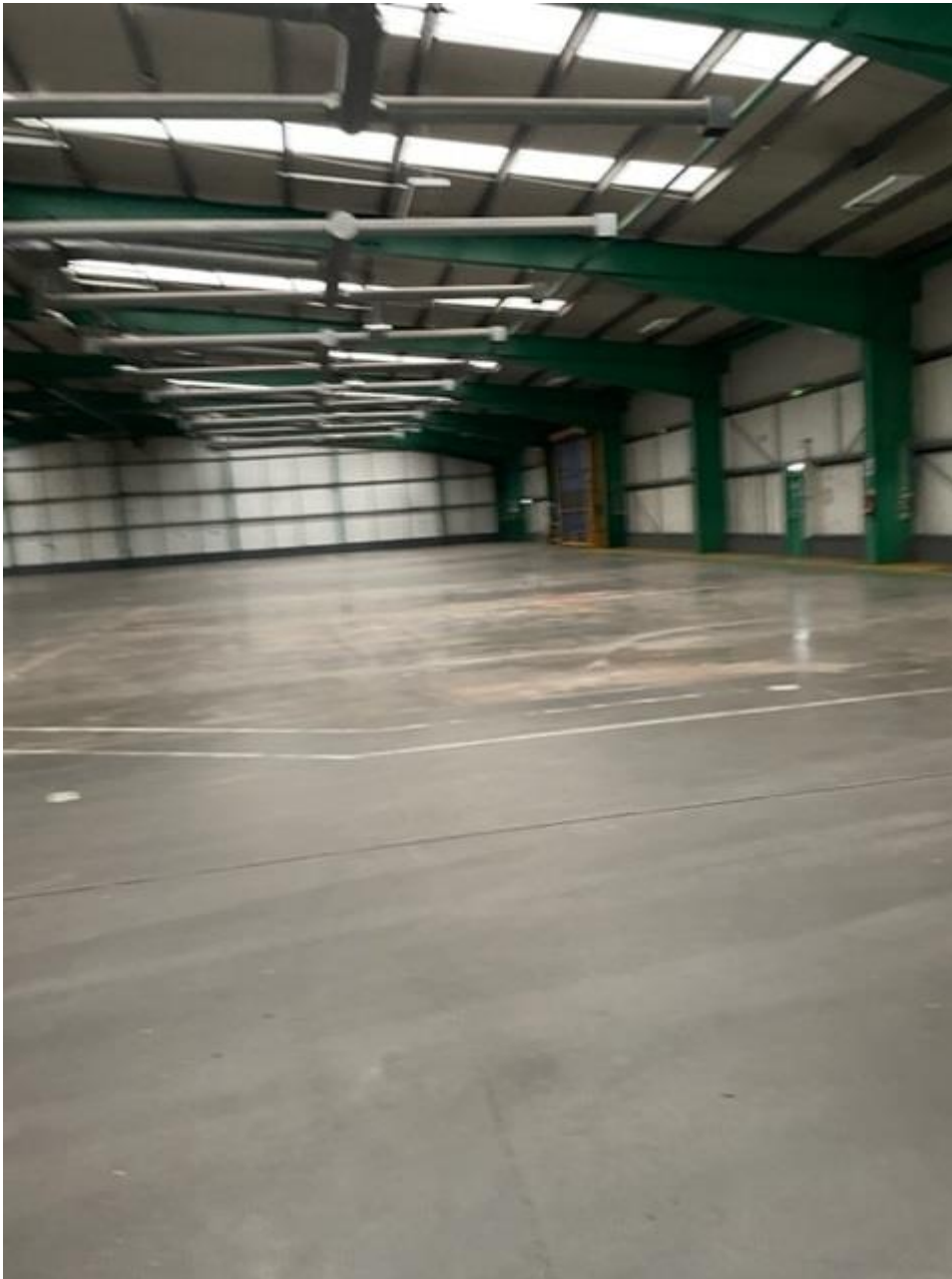
Inside storage shed – surfacing and infrastructure
