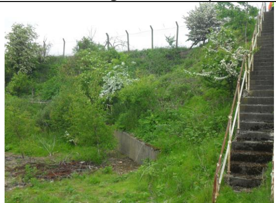
Detail of slope between area of former power station building and bases of the cooling towers
