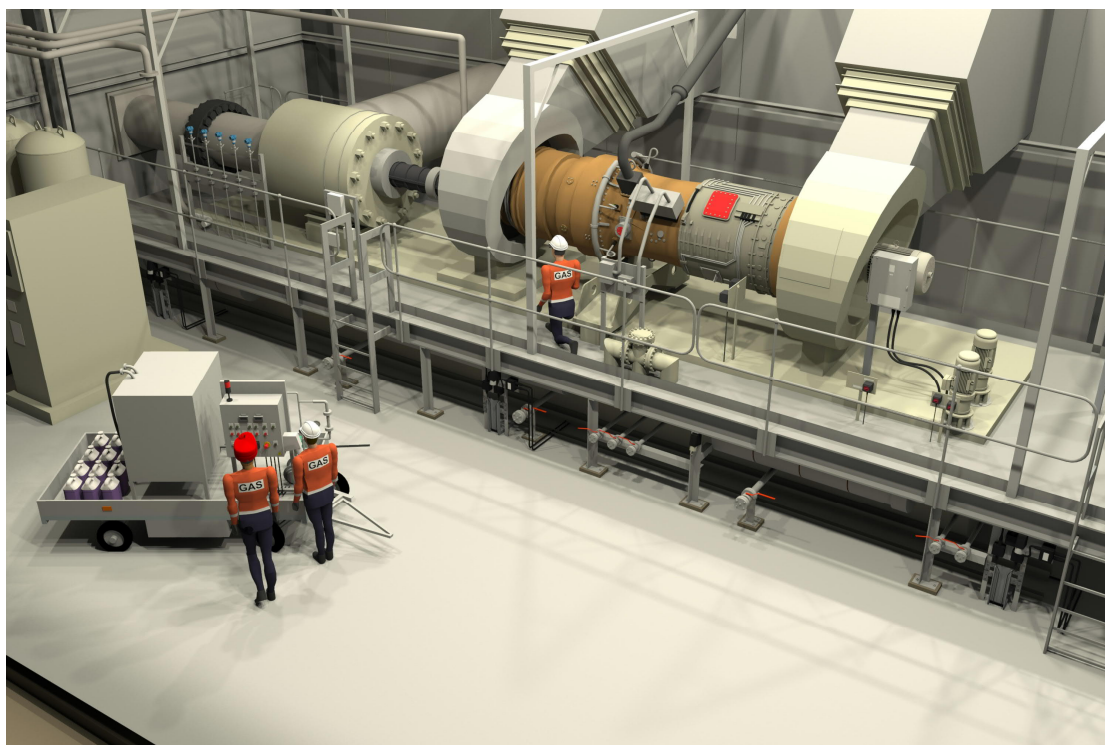
Figure I Conceptual illustration of turbine washing skid in a National Gas Transmission compressor enclosure
