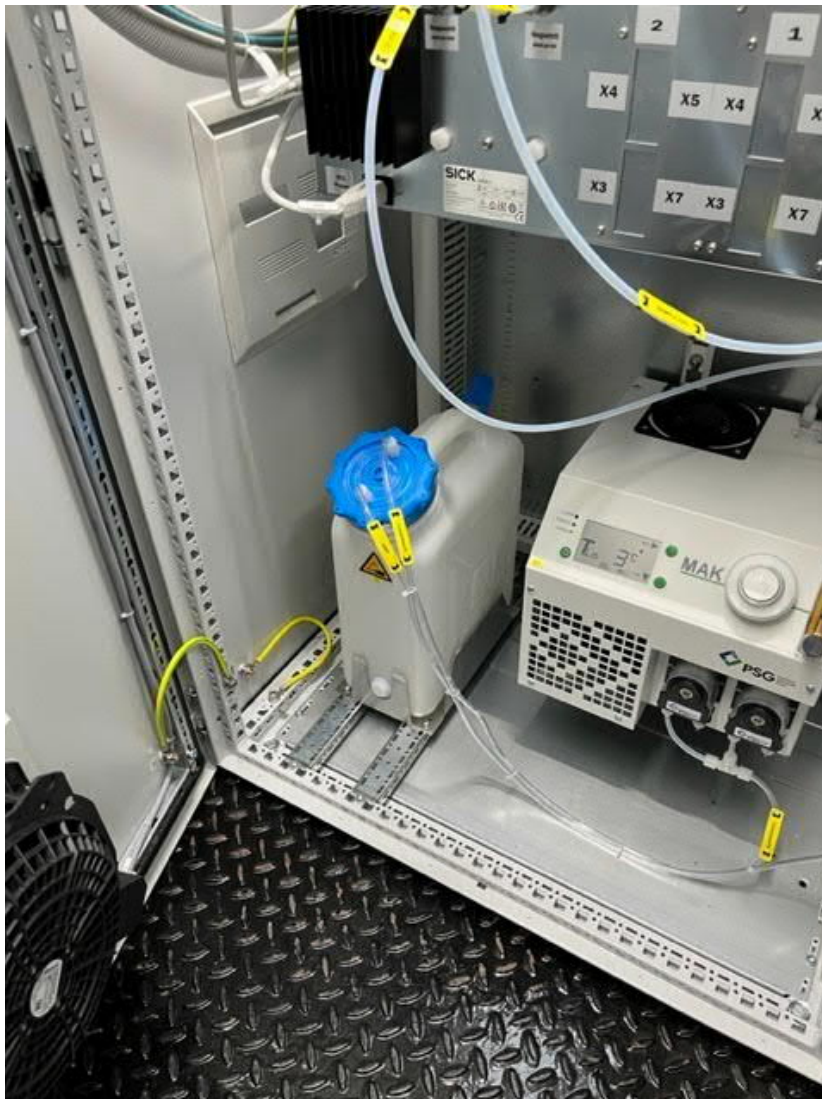
Figure J CEMS condensate collection in the Hatton enclosure
