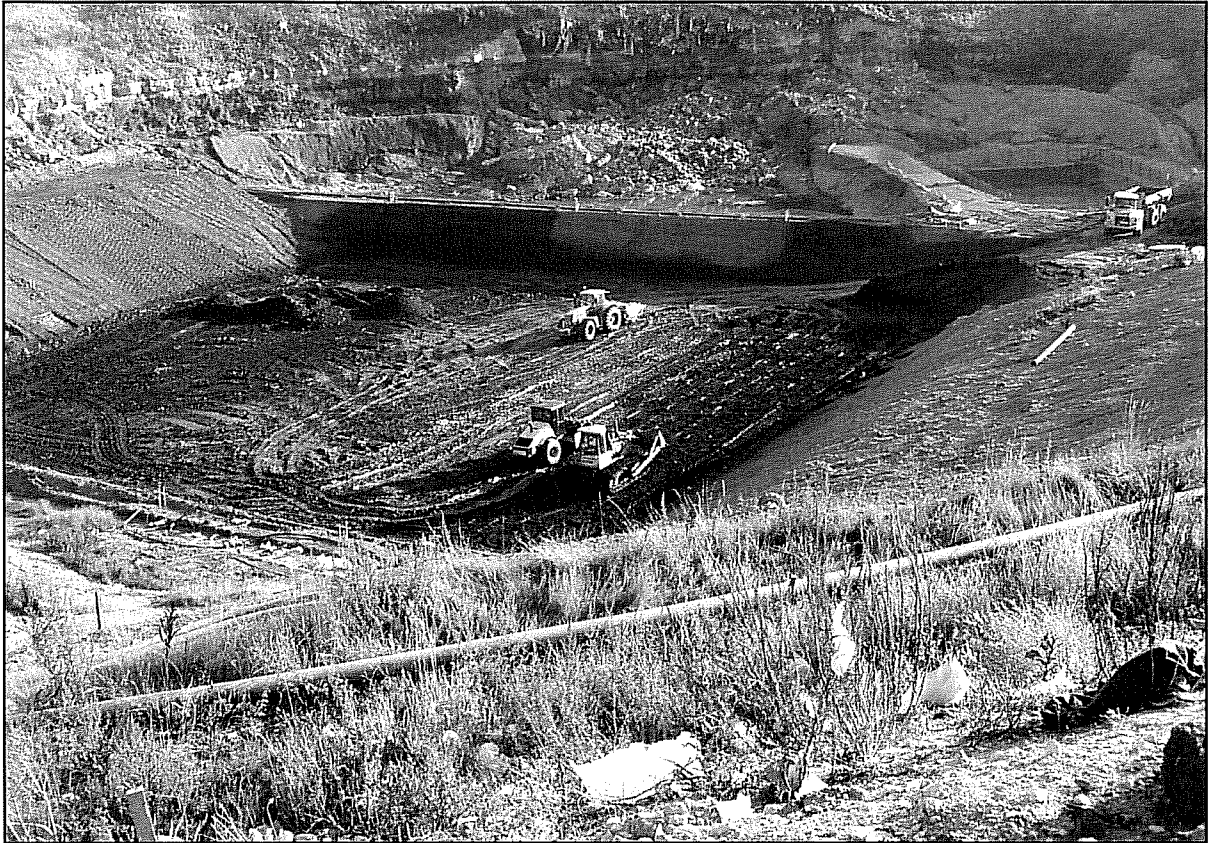
Plate 5 - Clay placement and compaction
