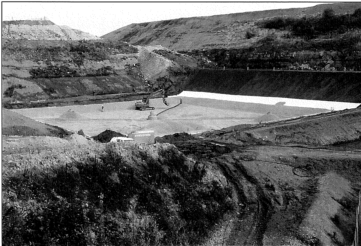
Plate 7 - Drainage blanket and leachate collection pipe work
