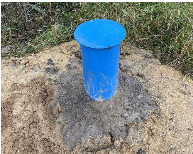
Figure 12 BH33 completed installation.
