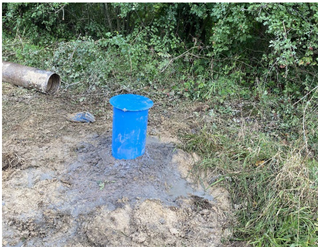
Figure 15 BH37 completed installation.
