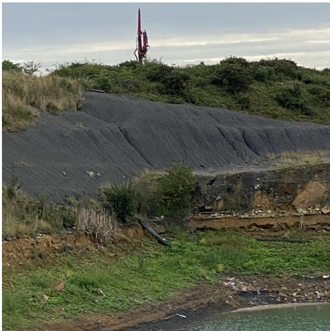
Figure 5 Site sidewall and rig set up at borehole location.
