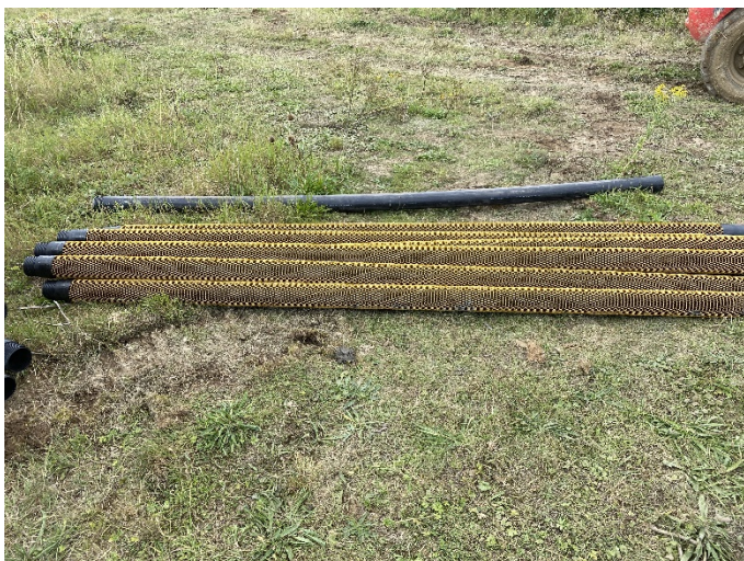
Figure 6 Slotted 3m pipework with pre-fitted geosock.
