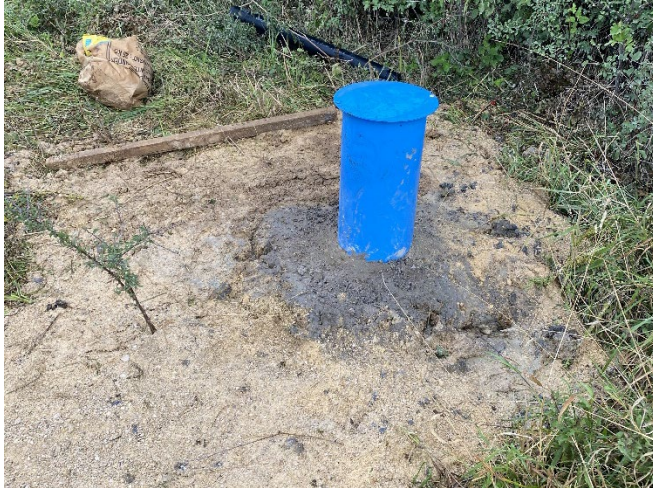
Figure 13 BH34 completed installation.
