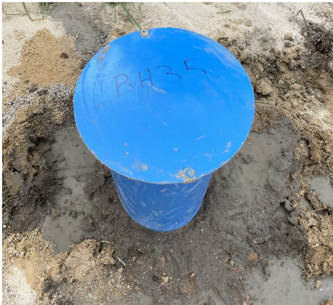
Figure 11 BH35 completed installation.
