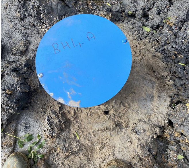
Figure 10 BH04A completed installation.
