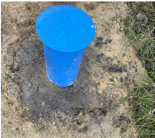
Figure 14 BH36 completed installation.
