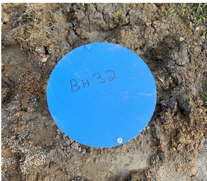
Figure 9 BH32 completed installation.
