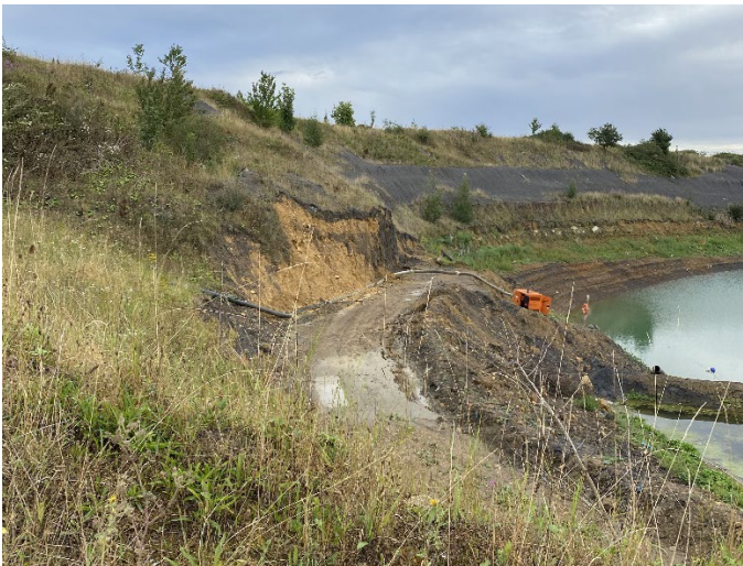
Figure 2 Site access and sidewall.
