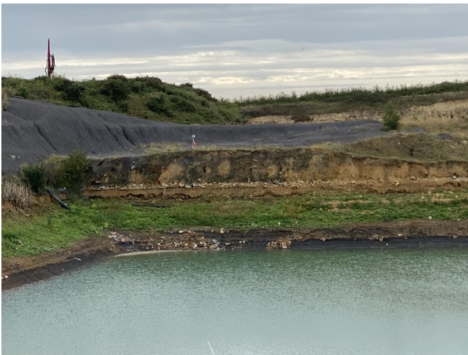
Figure 3 Site sidewall and rig set up at borehole location.
