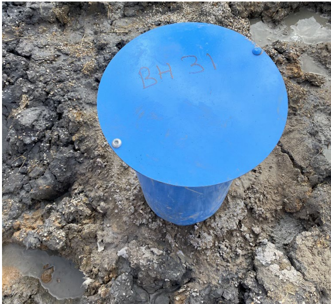
Figure 8 BH31 completed installation.
