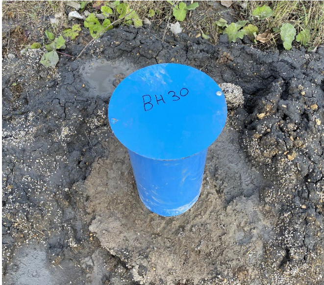
Figure 7 BH30 completed installation.
