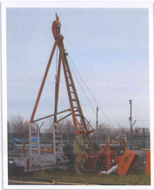
Photo 1. Cable Percussion Drilling Rig
