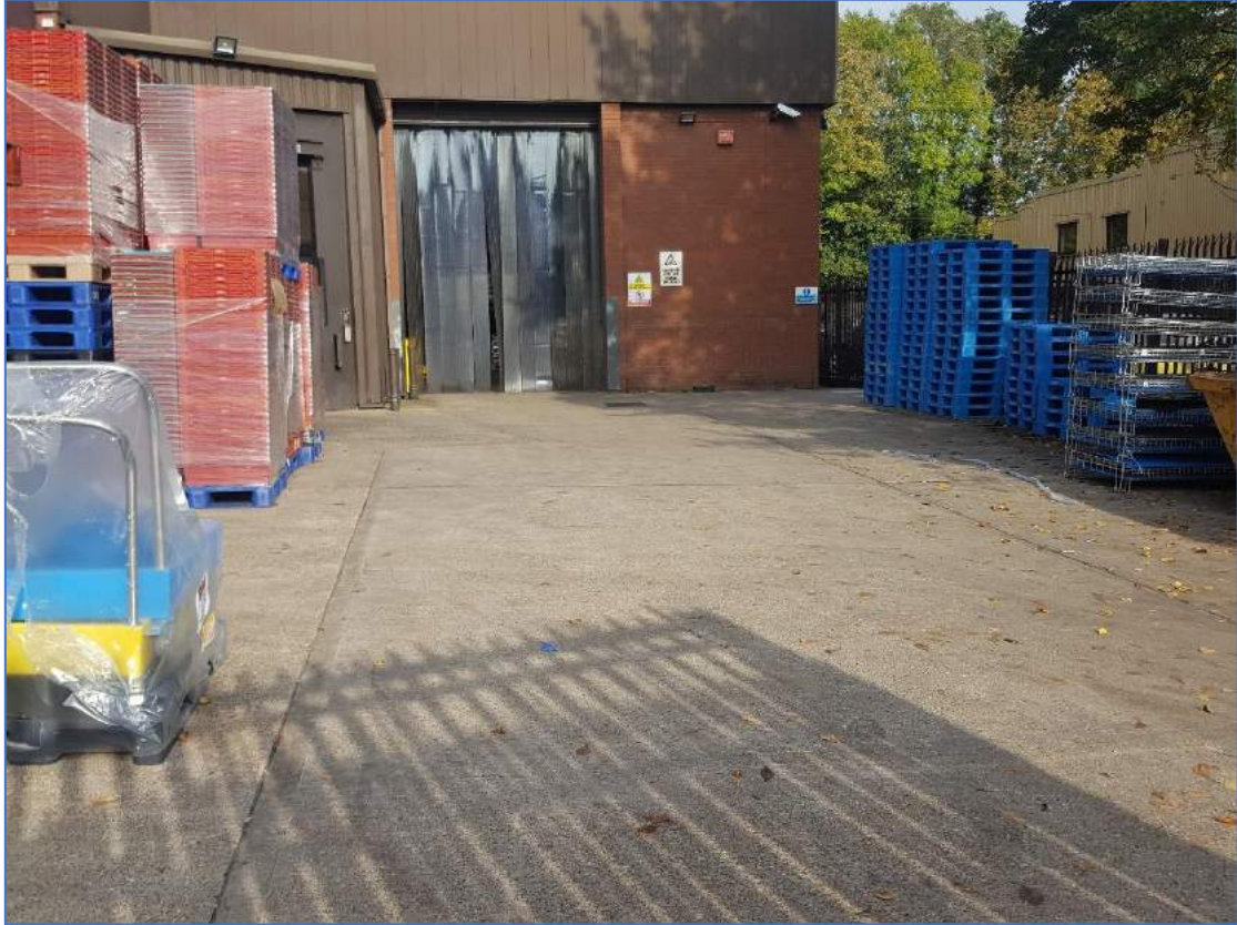
Photo 19 – Roller shutter doorway entrance to the raw materials warehouse
