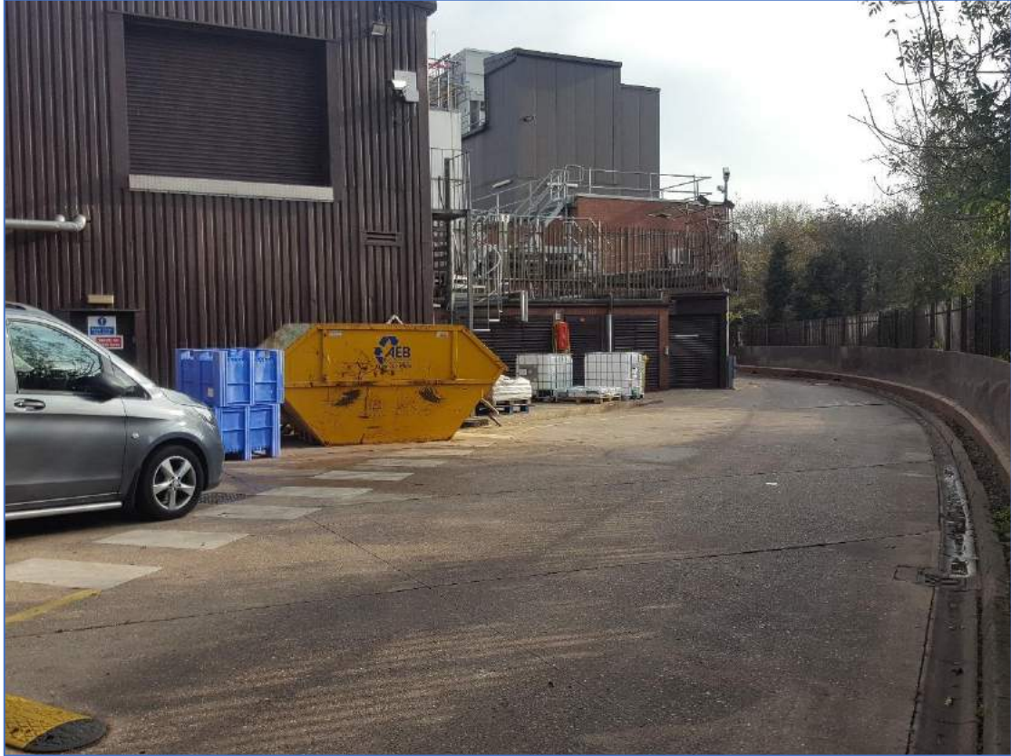
Photo 3 – Boiler house on the western perimeter of the production building
