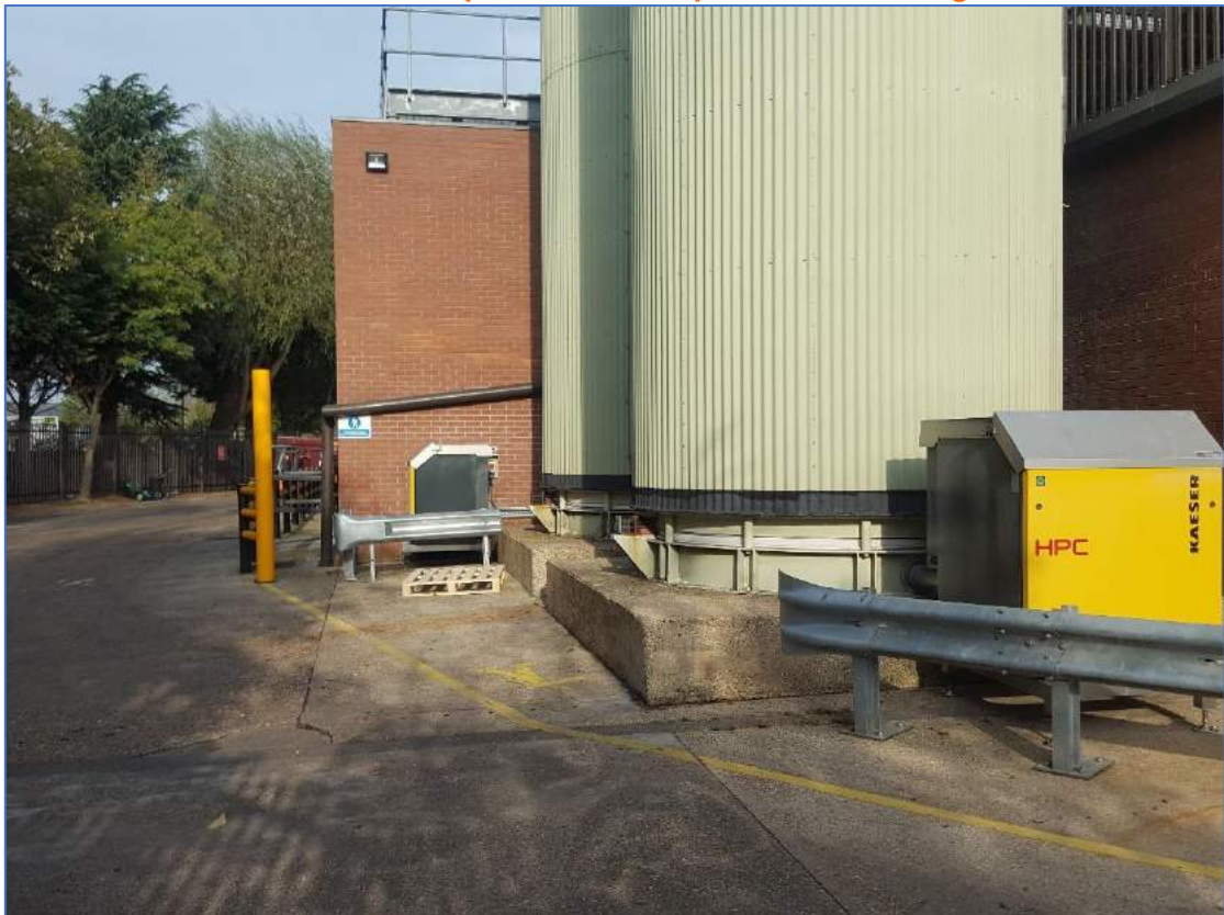
Photo 2 – Flour silos on the western perimeter of the production building
