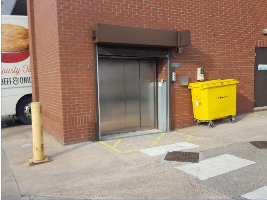
Photo 15 – Lower level lift shaft in the south eastern corner of the production building
