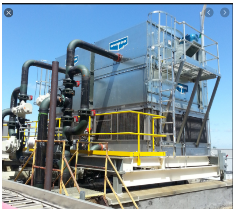
Figure 1: Typical Cooling Tower design
