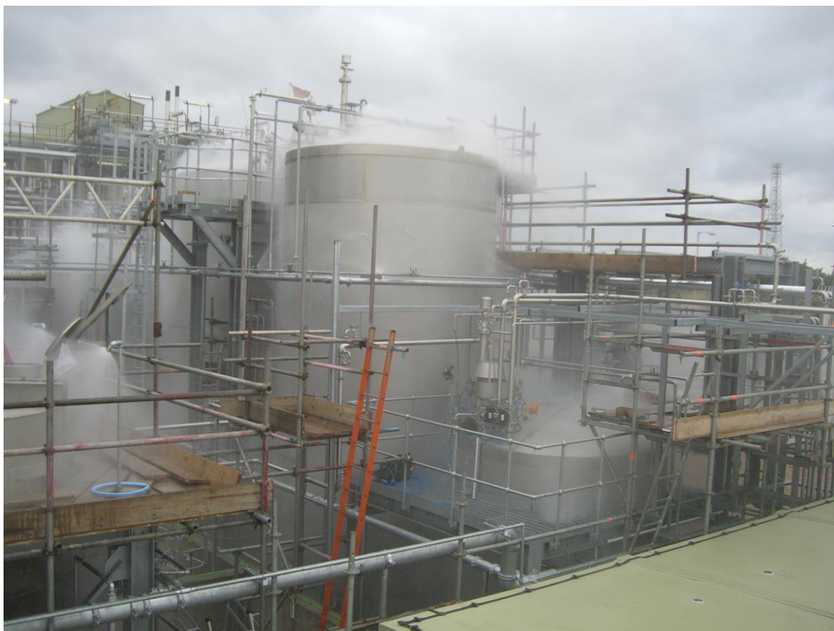
Typical tank farm in operation
