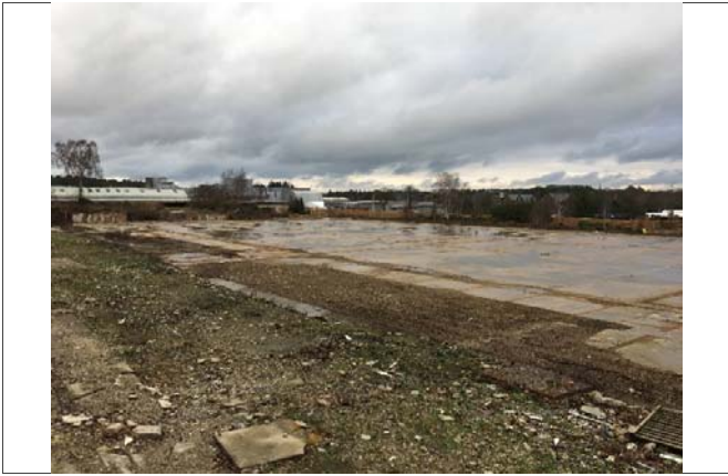
03: Central Slab Area
