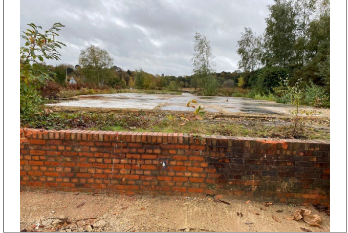
02: Low brick retaining wall
