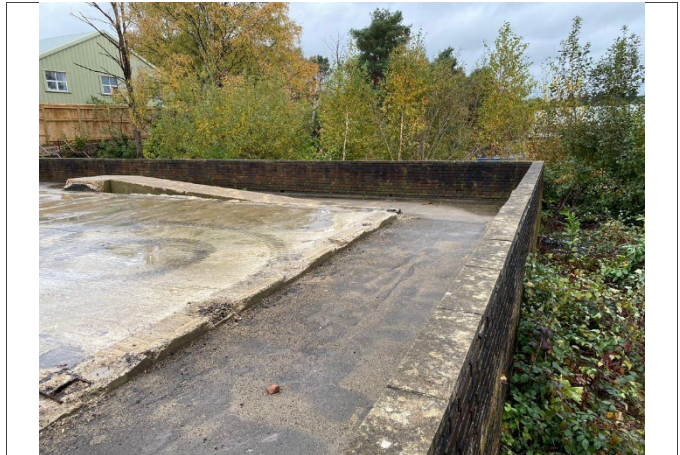
04: Raised concrete foundations
