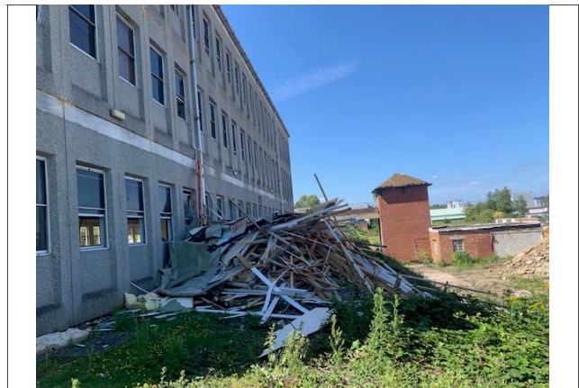
40: Constraints – Demolition stockpiles
