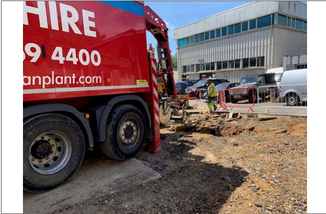
37: Constraints – vacuum excavation and deep excavations
