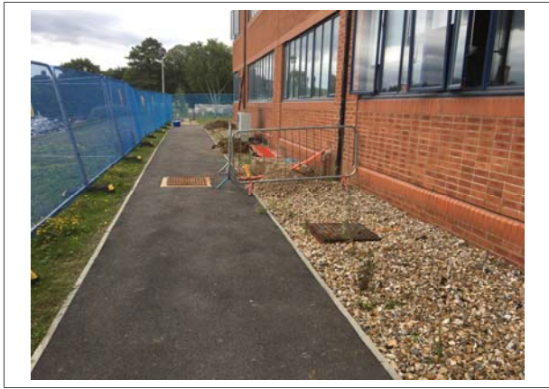
02: East wall of Building 124 facing south
