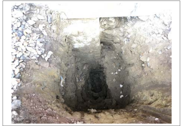
20: HDP4 right of drain
