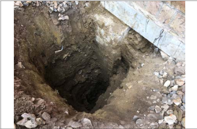
19: HDP4 right of drain
