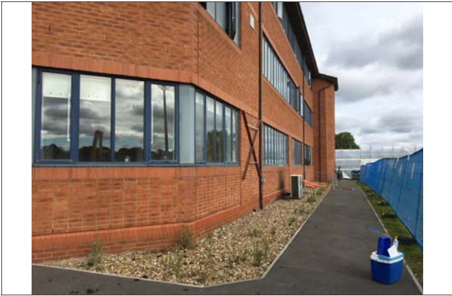
01: East wall of Building 124 facing north
