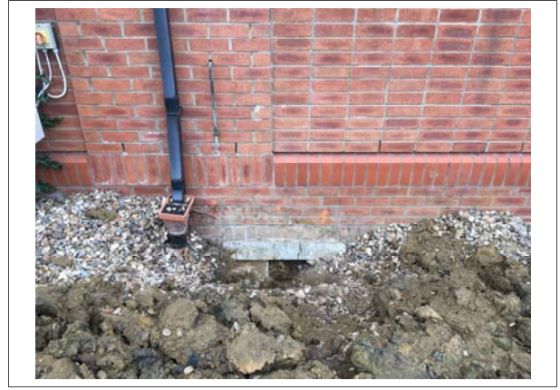
18: HDP4 right of drain
