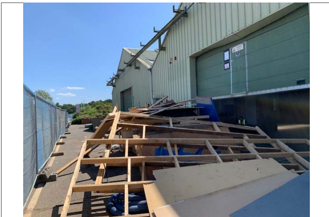
39: Constraints – Demolition stockpiles
