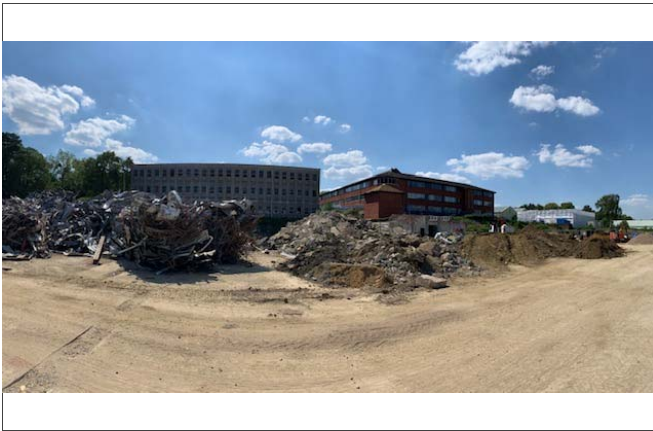
43: Constraints – Demolition stockpiles and vehicular access
