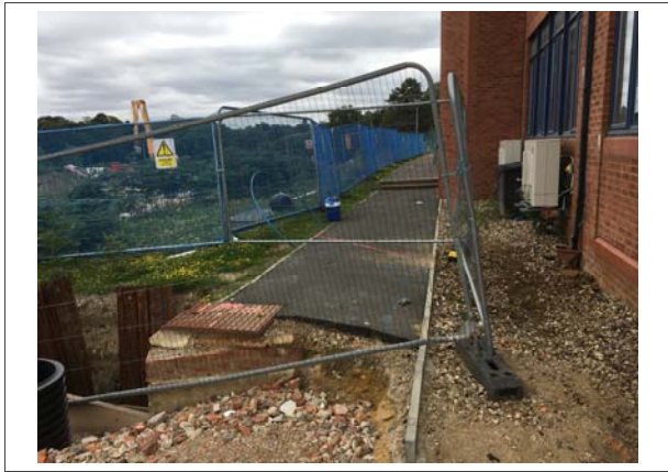
04: Northern part of Building 124 facing south
