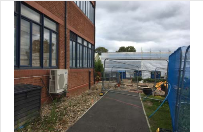
03: Northern part of Building 124 facing north
