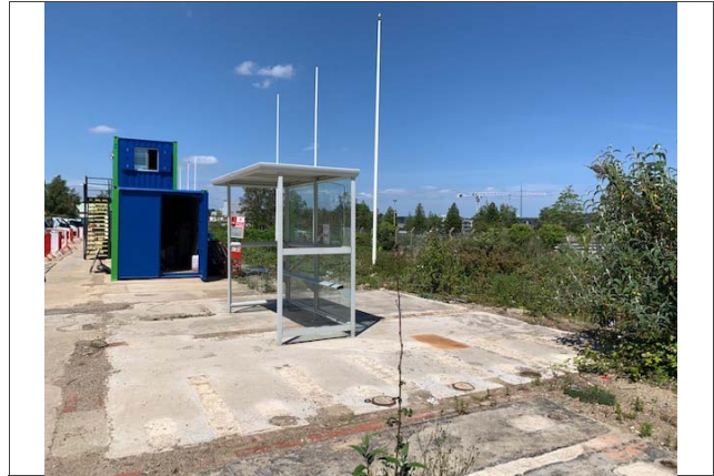
38: Constraints – site cabins / set up
