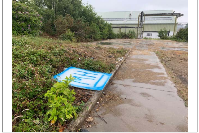
06: Hardstanding of building 60/61
