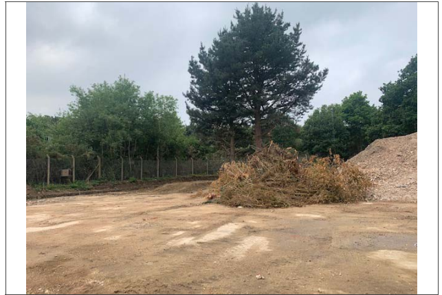
08: Former Canteen (Building 100, 101)
