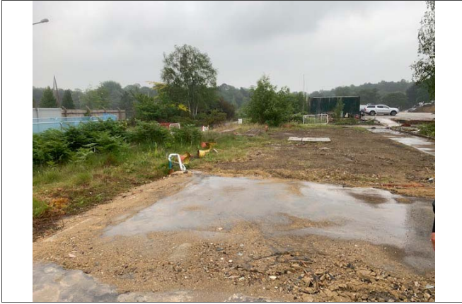
05: Hardstanding of building 60/61
