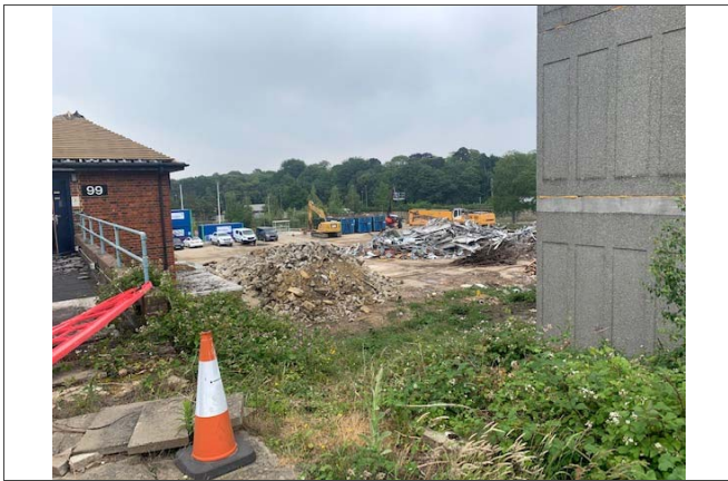
03: View from the top of the slope (southeast)
