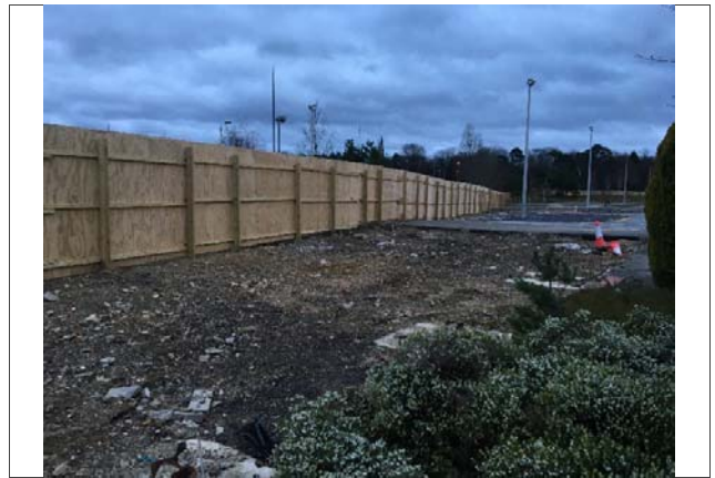
12: Northern Part of the site
